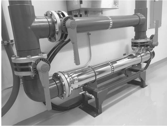
FIGURE 24.3 UV sanitization. An example of a UV sanitizing unit for aquaculture.
