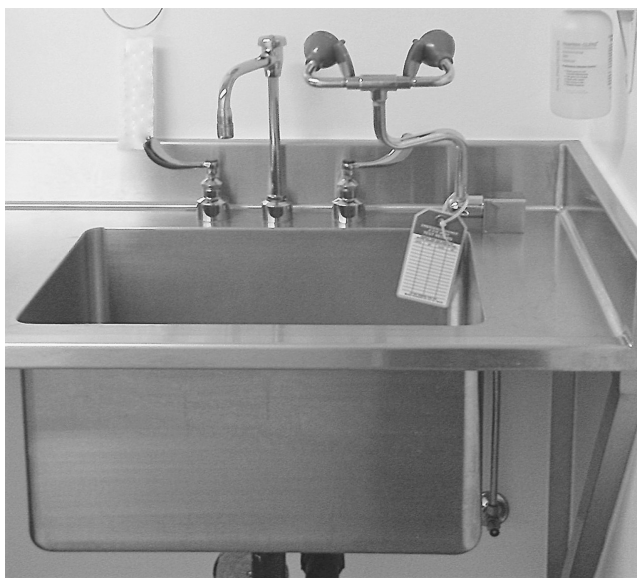
FIGURE 26.13 Eyewash station with card for documenting when station was tested. (Photo by Michelle Wallace-Fields.)
