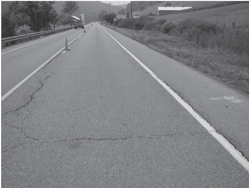
Figure 20. Transverse and longitudinal cracks on PG 64-22 section of the clearfield project.
