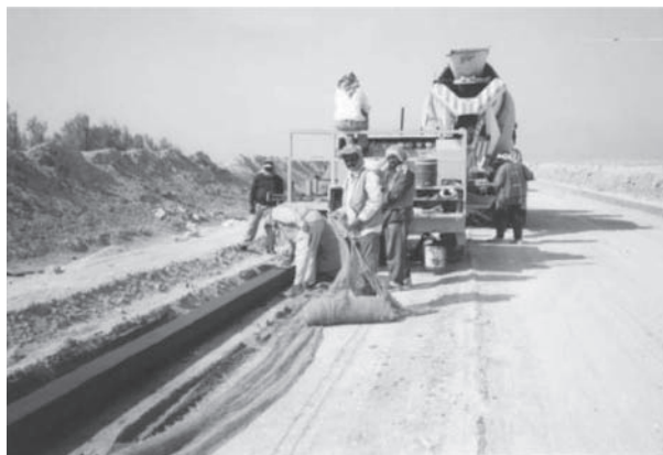
Figure 3. Construction of sunken concrete curb.
