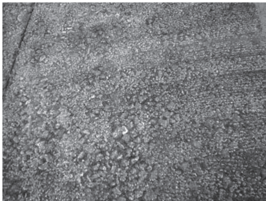
Figure 5. Surface of the base layer after fine milling.
