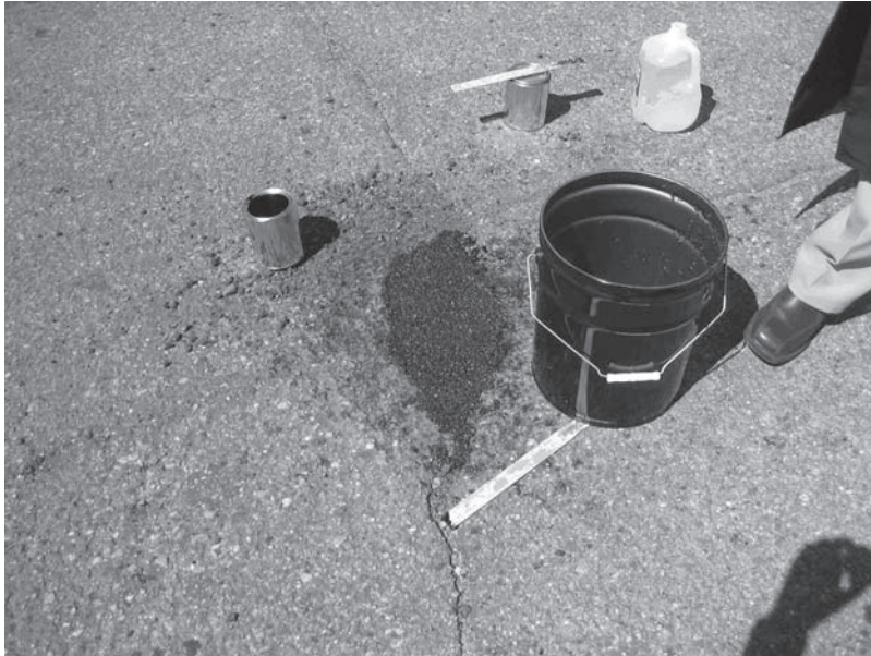
Figure 5. Trial lay down For PMA with carrier and PT-743.
