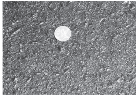
(a) Compacted Using AMIR Roller
