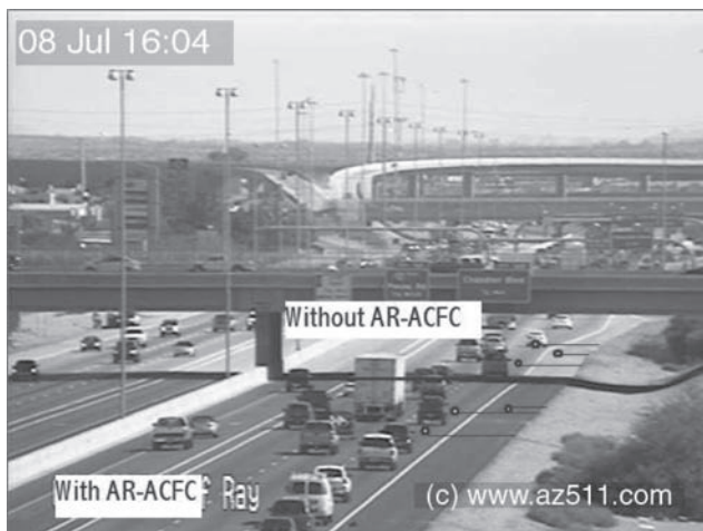
Figure 6. Ray road test site at I-10.
