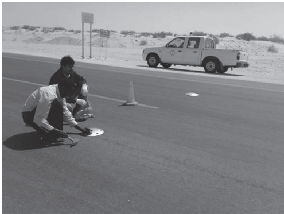
Figure 2. Installation of traffic counters on Khursaniyah access road.
