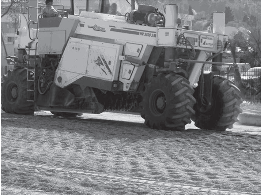
Figure 2. Implementation of the CIR technique using foamed asphalt.
