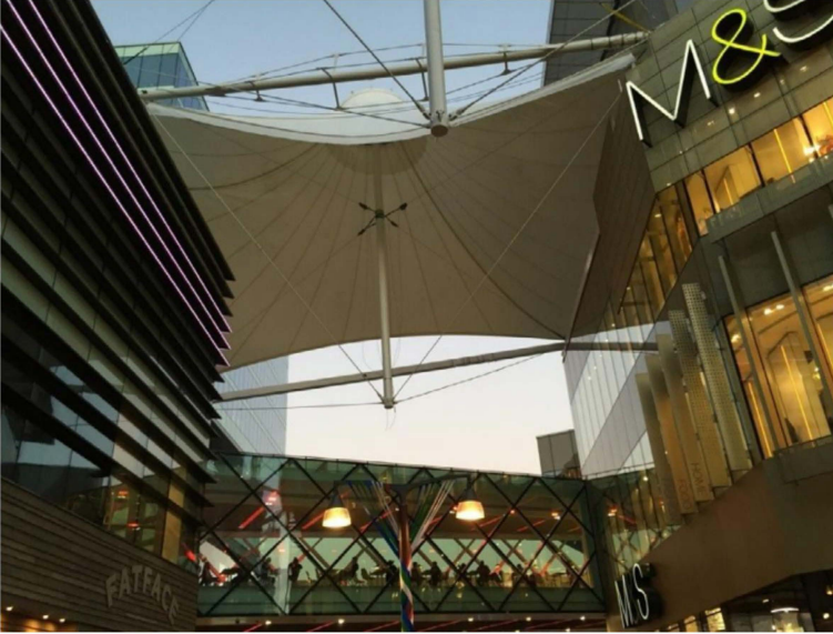
Fig. 7.15 Unit tensegrity structure in Westfield Shopping Center, Stratford, London, U.K. (Photo taken by the author.)
