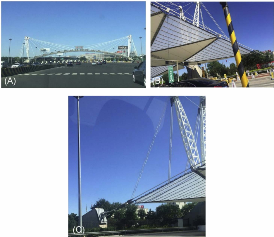
Fig. 7.2 A tensile membrane canopy of a toll station at Highway of Beijing International Airport, Beijing, China: (A) overview of the entire structure, (B) details of mast connection to concrete foundation support, and (C) details of cable support. (Photo taken by the author.)
