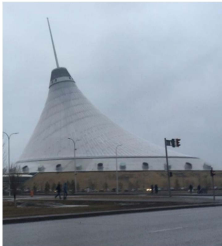
Fig. 7.3 Membrane structure Khan Shatyr Entertainment Center, Astana, Kazakhstan. (Photo taken by the author.)
