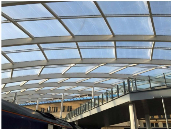
Fig. 7.5 Membrane roof in Manchester Victoria Train Station, Manchester, UK. (Photo taken by the author.)
