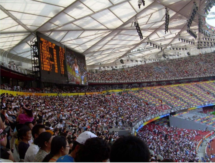
Fig. 7.10 Membrane roof of Birds Nest Stadium in Beijing, China. (Photo taken by the author.)
