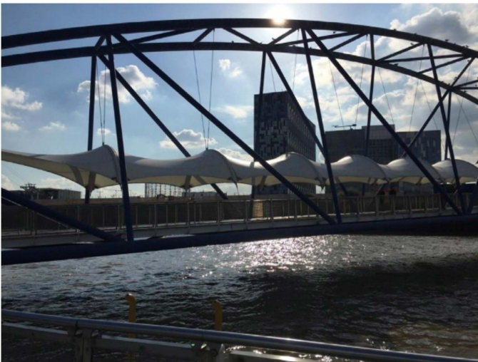
Fig. 7.7 A bridge with arch supported membrane canopy at Greenwich, London, UK. (Photo taken by the author.)
