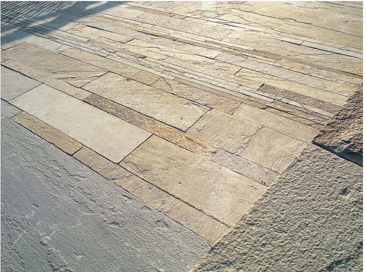
Upper level, bluestone paving
