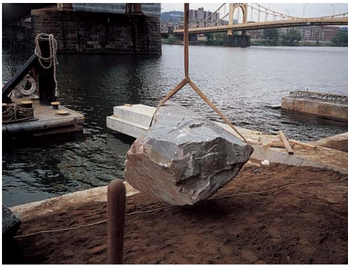
LEFT: Large chunks of bluestone individually placed between cantilevered walkway beams RIGHT: Use of smaller liner stock trees allows close spacing of trees between stones
