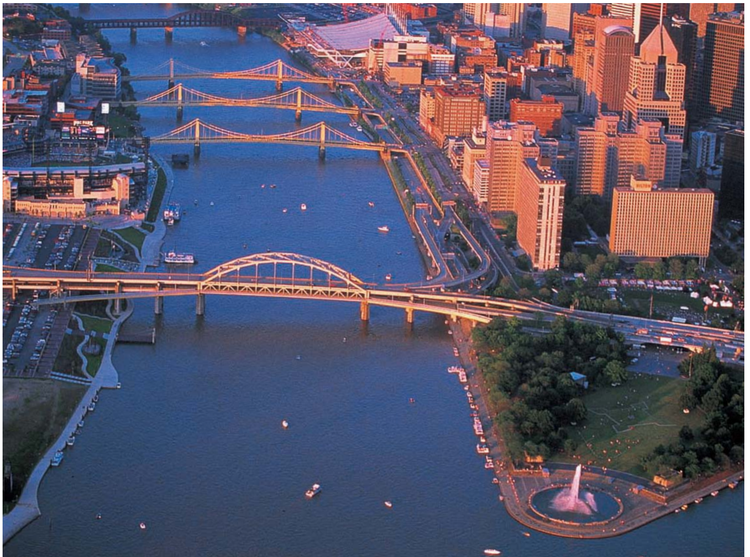
Aerial view of site with Point State Park in foreground
