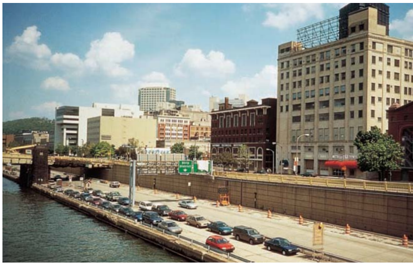
Existing site conditions in 1994, showing the topographic division that creates the lower and upper levels of the park and the highway and seawall
