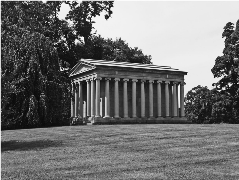
FIG. 6.3. Jay Gould's Mausoleum from the southeast. E. Macaulay-Lewis.
