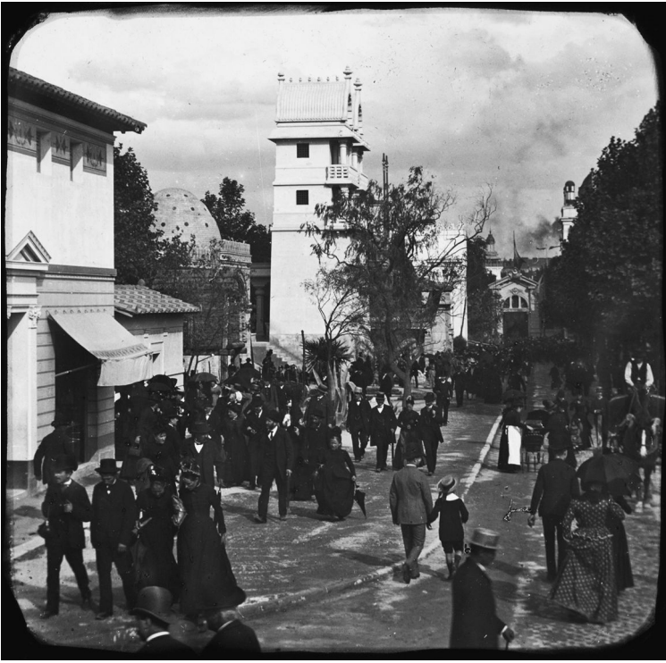
FIG. 3.1. View of L'Histoire de l'habitation humaine exhibition from the corner of the Roman House (N.B. This is an inverted image).
