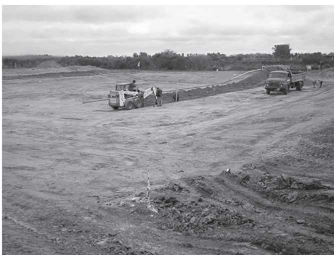
Figure 2. Waterproofing of the wetland area using bentonite.
