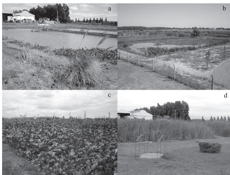
Figure 4. Stages of vegetation development in the constructed wetland: (a) during transplantation, where the baffle is observed; (b) 4 months after transplantation; (c) one year of operation (dominance of floating species); (d) after three years, where the dominance of emergent species and the income of the effluent pipe is observed.
