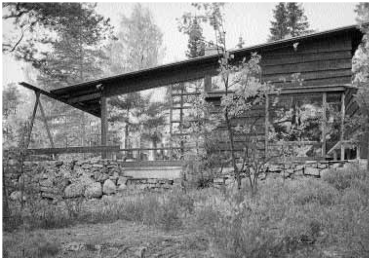
Single-family house with photo atelier on Gråkamveien
