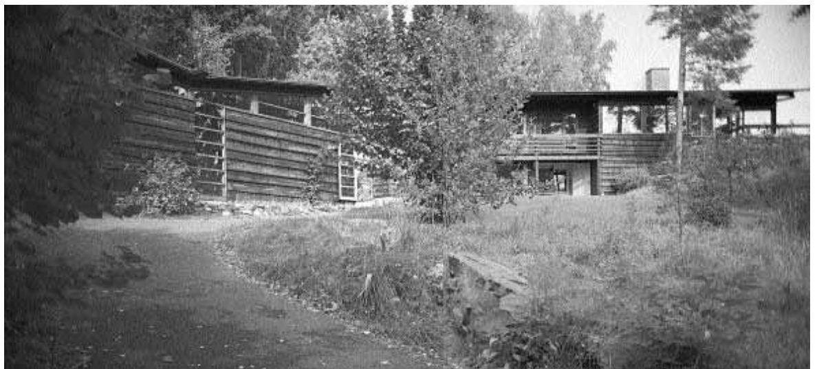
Single-family house with photo atelier on Gråkamveien
