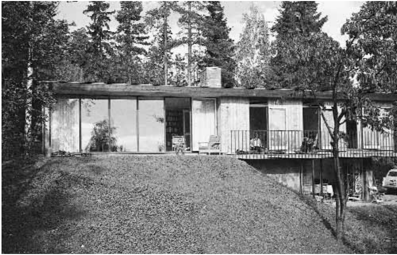
Single-family house in Besserud
