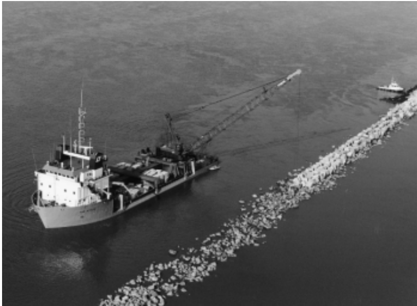
Figure 13-22 Placing elements on a breakwater with crane ship (van Oord ACZ)
