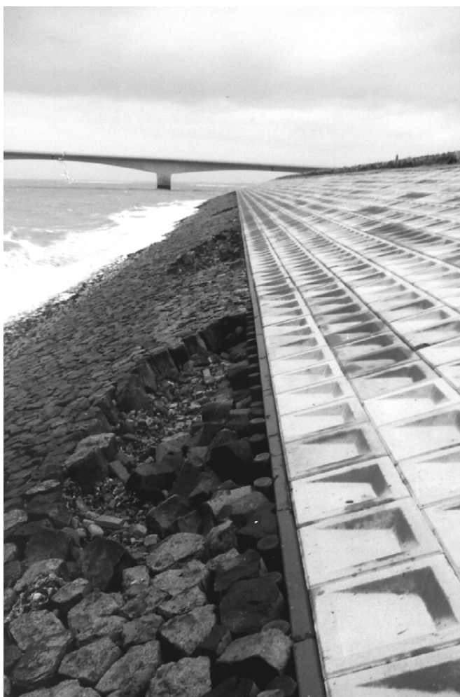
Dike with basalt columns and concrete blocks (Zeeland), courtesy Rijkswaterstaat
