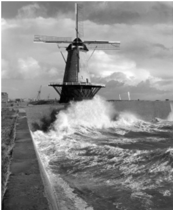
Figure 11-27 Seawall Flushing (photo Wil Riemens, Middelburg)
