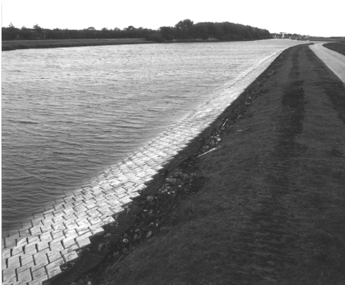
Figure 11-17 Block mat as bank protection
