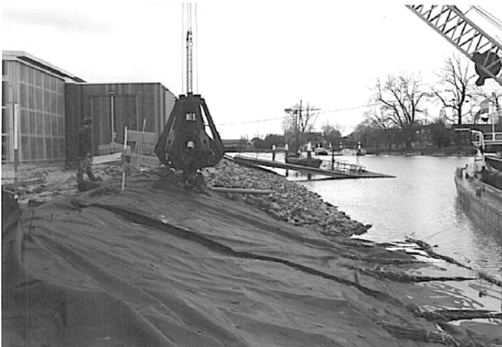
Figure 13-13 Placing stones with floating crane and grab (Johan van der Ham)
