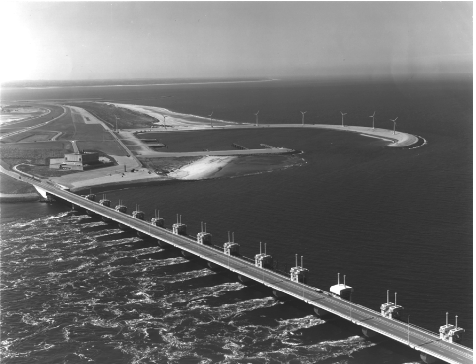
Outflow Eastern Scheldt storm surge barrier (courtesy Rijkwaterstaat)
