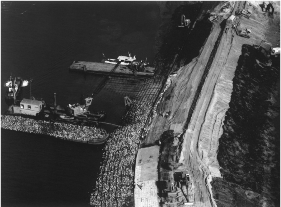
Figure 13-14 Placing fascine mattress on revetment
