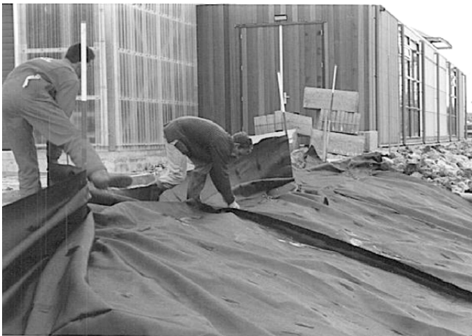
Figure 13-11 Placing geotextile in simple revetment (Johan van der Ham)
