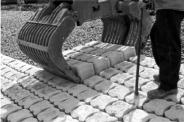
Figure 13-18 Mechanical placement of Hydroblocks (courtesy Greenbanks)
