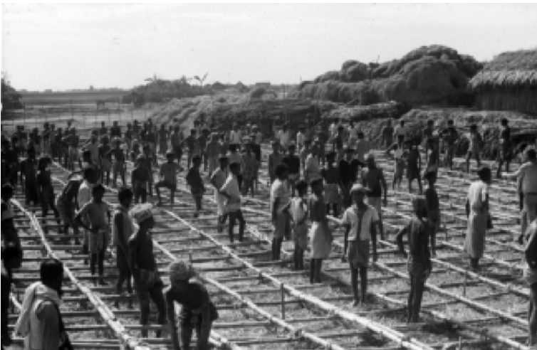
Figure 13-9 Construction of bamboo mattress
