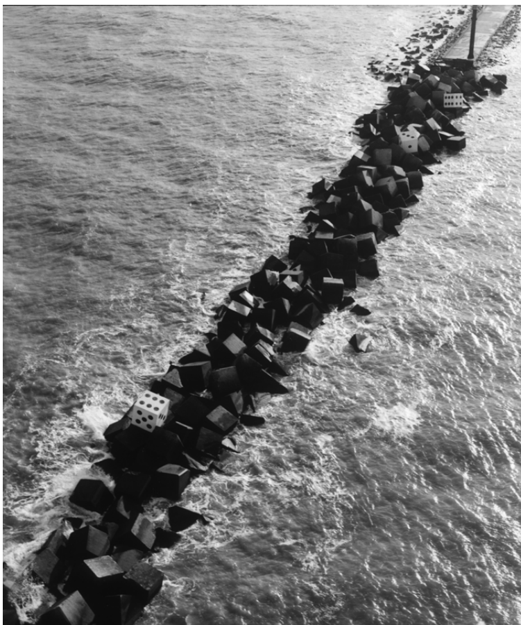
Dice blocks on breakwater Hook of Holland (courtesy Rijkswaterstaat)
