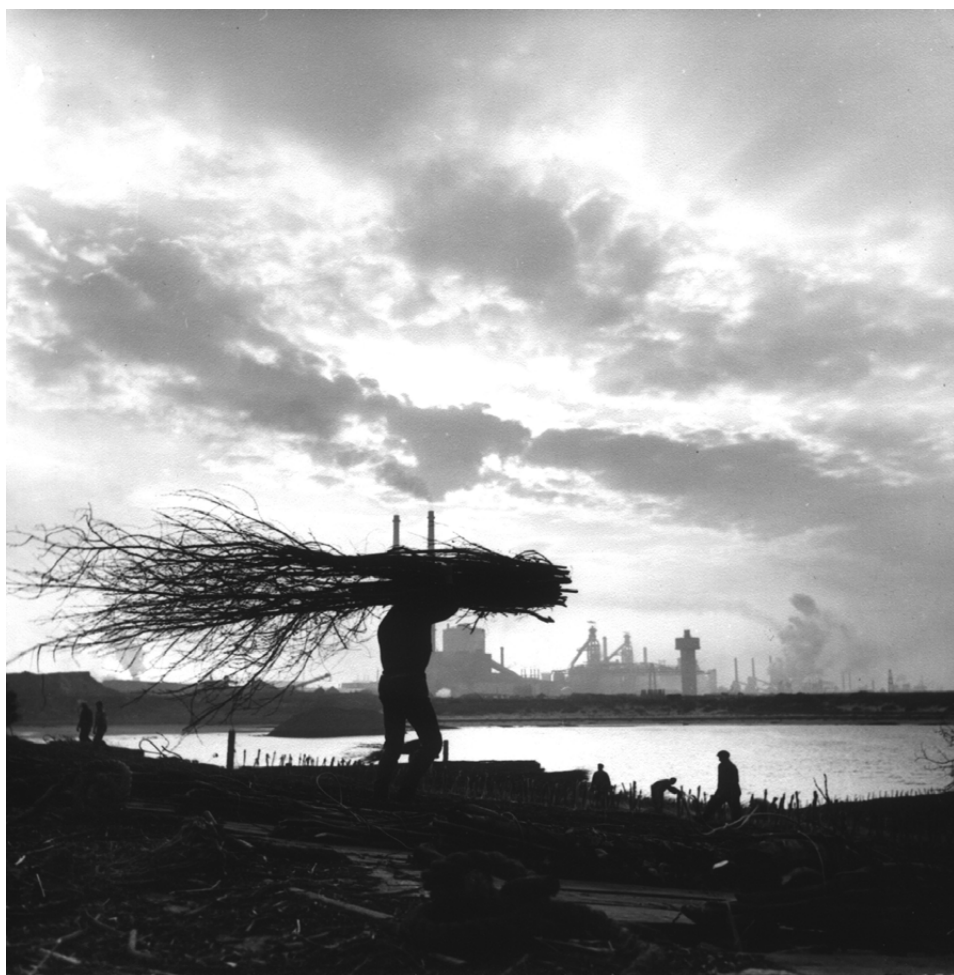
Brushwood for the construction of a mattress
