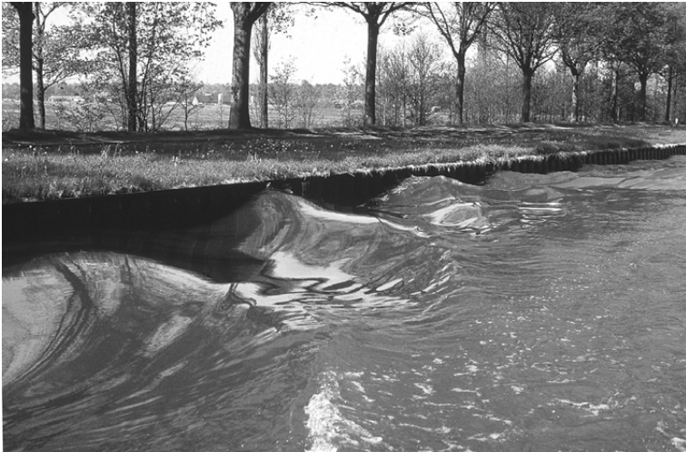
Figure 11-18 Sheet pile wall along canal (CUR 200, 1999)
