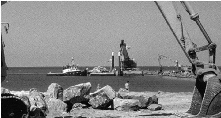
Figure 13-20 Construction of a groyne using both land based and marine equipment
