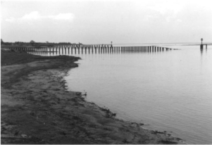
Figure 11-22 Pile screens in Jamuna river Bangladesh
