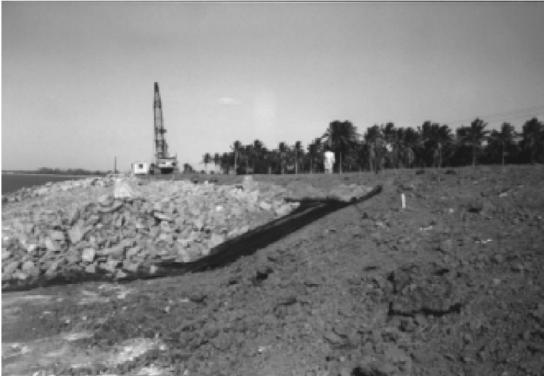
Figure 11-23 Loose rock dike revetment (Nickerie, Surinam, Leo Philipse)
