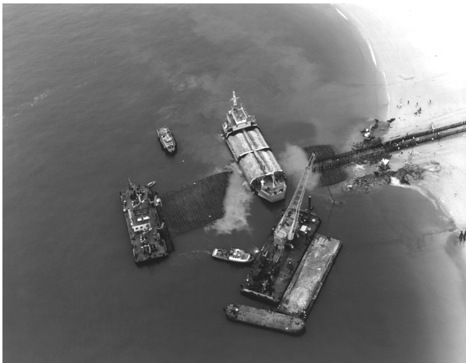
Construction of beach groyne (courtesy Boskalis)
