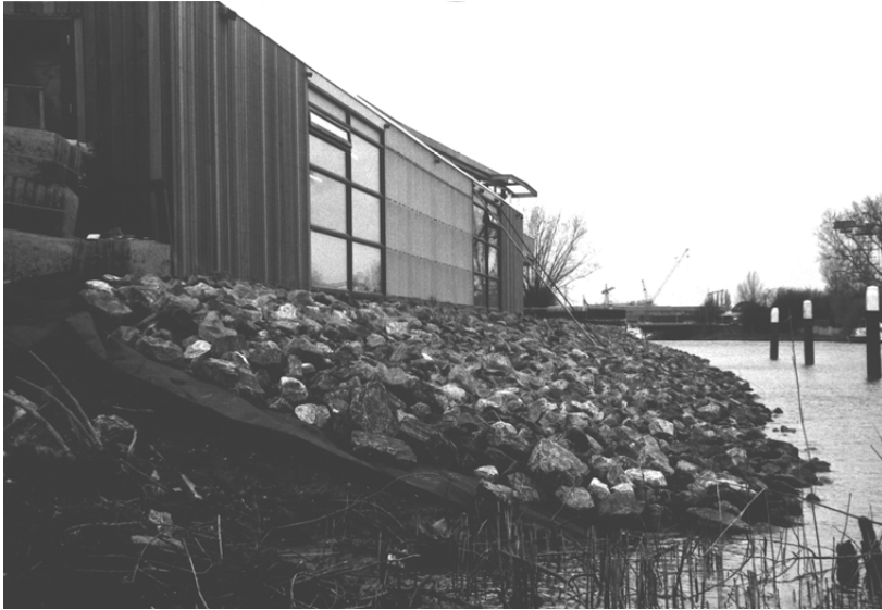
Figure 11-16 Simple bank protection with geotextile
