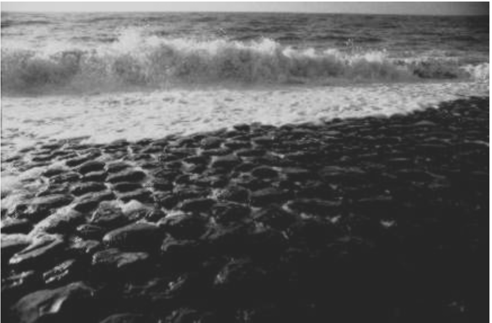
Spilling breaker on dike slope (Zealand)
