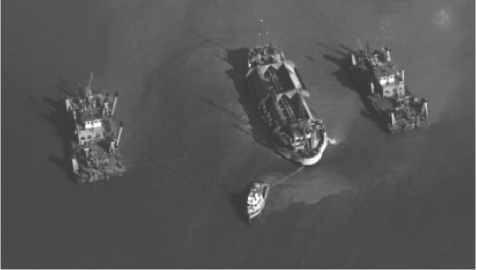
Figure 13-8 Sinking fascine mattress
