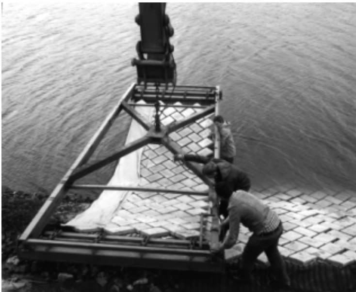
Figure 13-16 Placing of prefabricated mat on revetment
