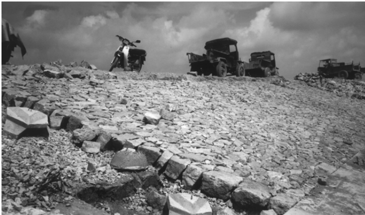
Figure 11-24 Placed block revetment (Vietnam)
