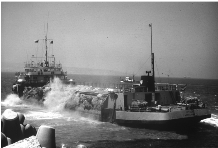
Figure 13-5 Side stone dumping vessel (courtesy Boskalis)
