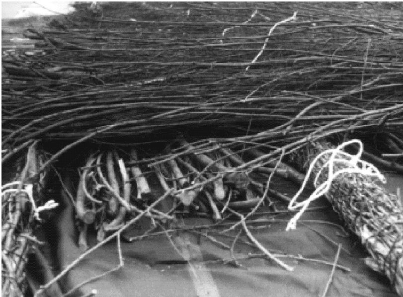
Figure 11-8 Geotextile under mattress
