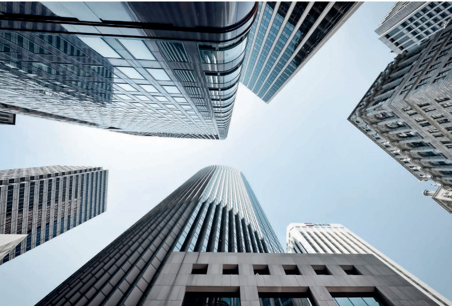
Fig. 255: Large areas of sky set the stage for the receding skyscrapers in this overhead shot [focal length: 14mm]
