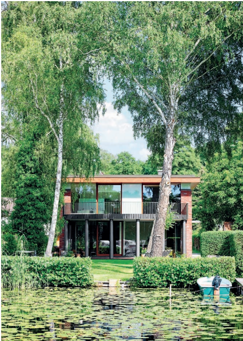
Fig. 161: Elements of the surroundings influence the overall impression made by a building
