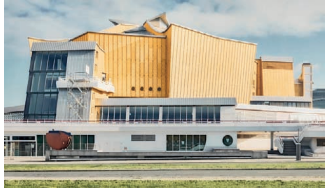
Fig. 173: The same building, photographed later
