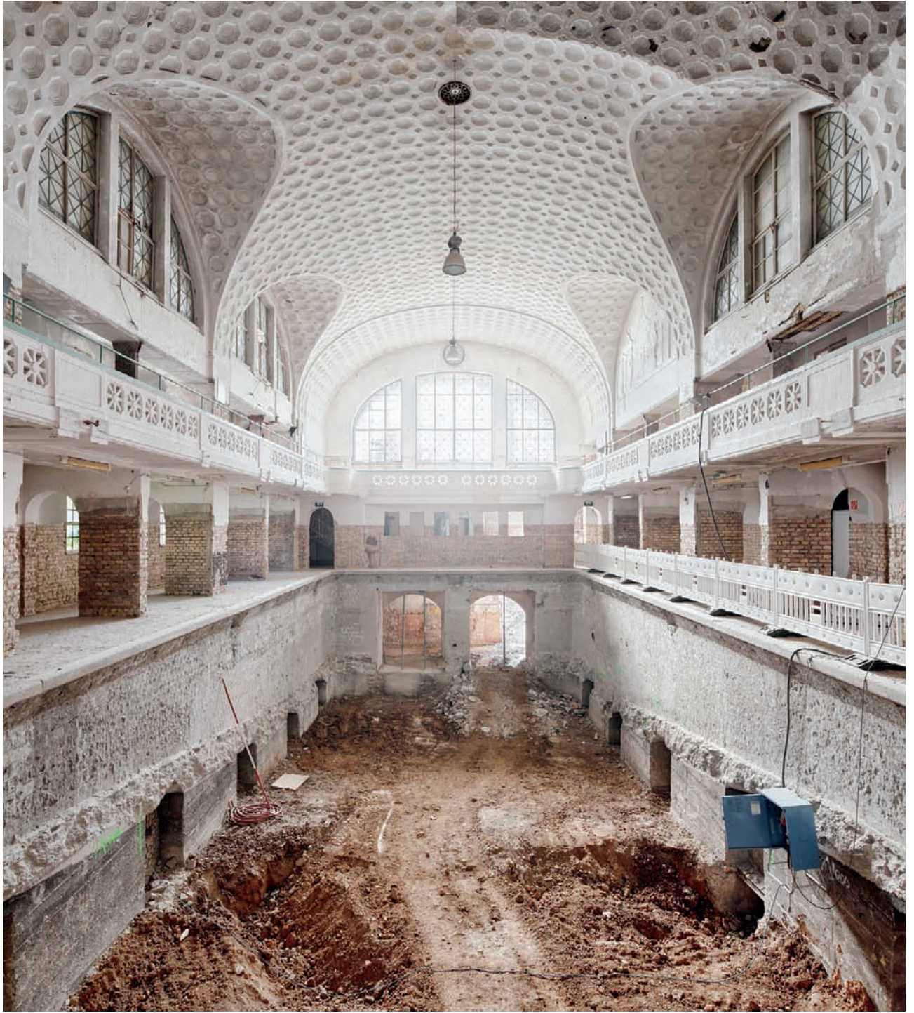
Fig. 218: This image was exposed for the interior, which in turn causes the window areas to appear excessively bright as a result of the marked contrast
