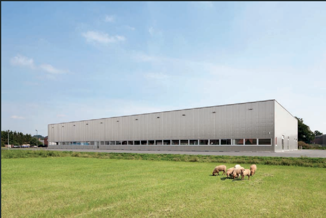
Fig. 269: Warehouse, Osnabrück; photo: Marcus Bredt
