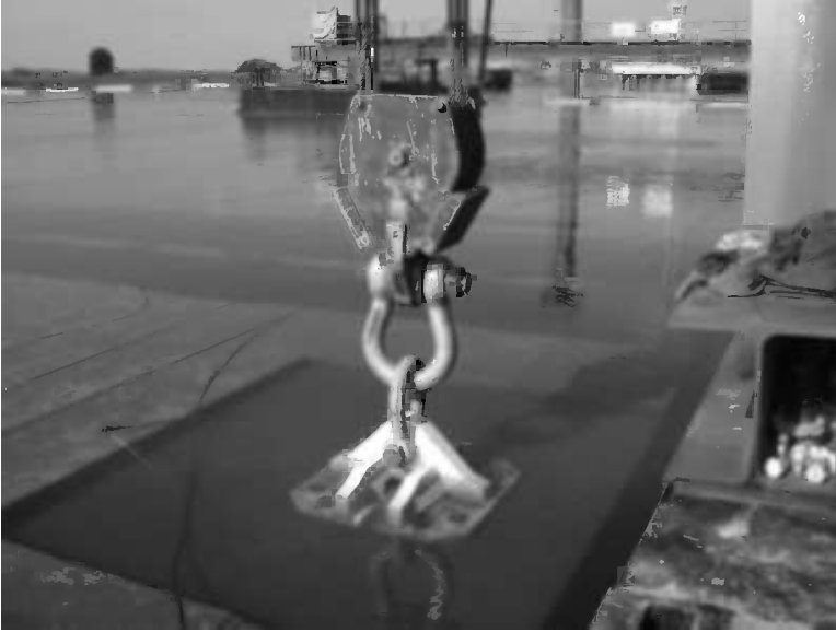
Figure 14.14 Typical suspension lug with lowering winch cable attached. (Photo courtesy of Strukton.)
