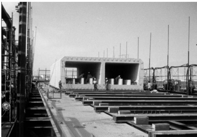
Figure 14.9 Tunnel element assembly on ship lift in Tuas Bay.
