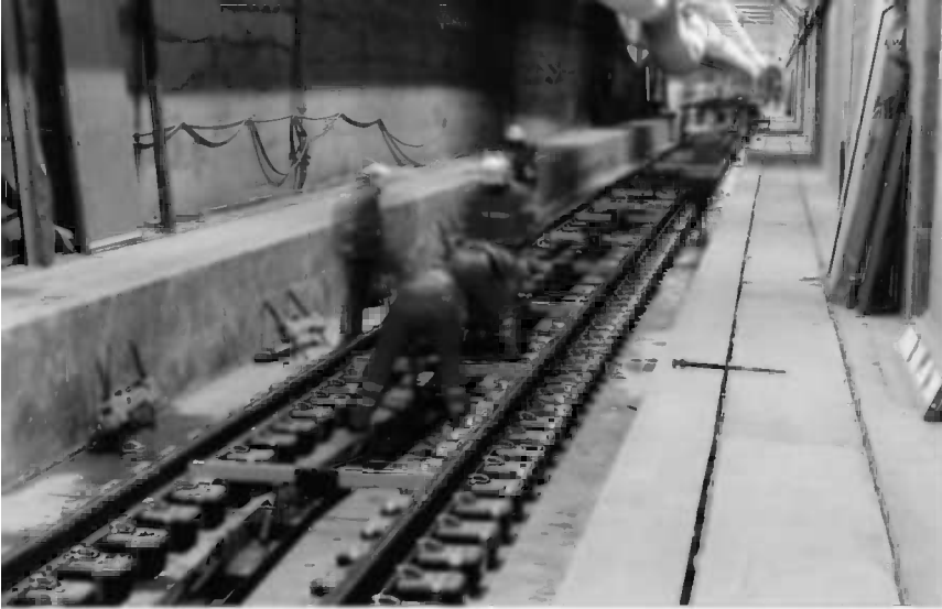
Figure 15.6 Fixing booted track system in the Øresund Tunnel. (Courtesy of Øresundsbron.)
