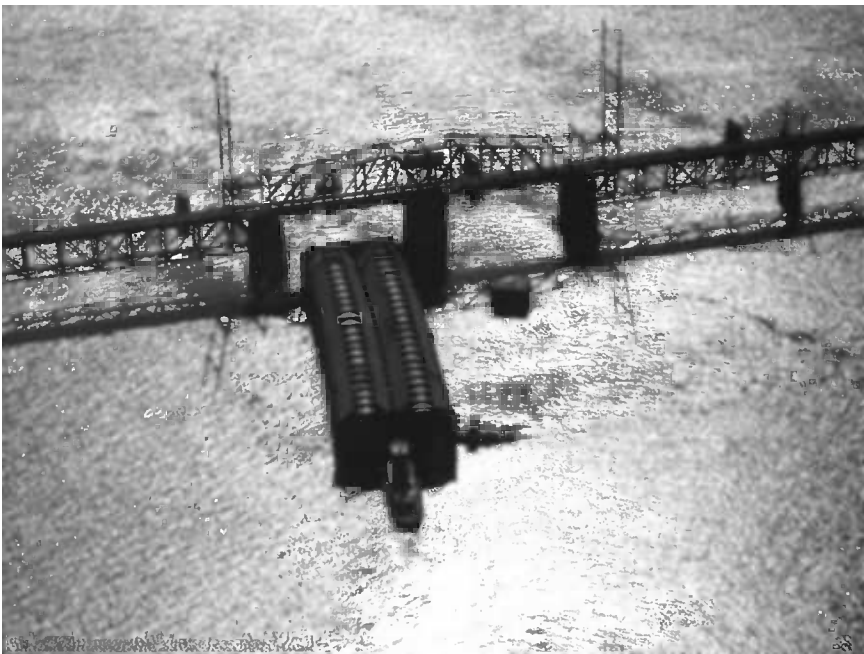
Figure 14.24 Steel shell element being transported. (Photo courtesy of W. Grantz.)
