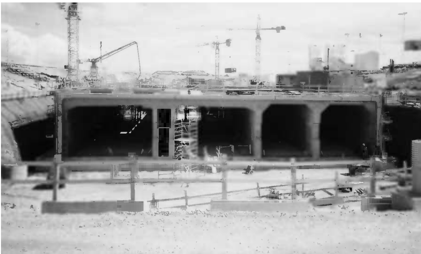
Figure 8.2 Cut and cover tunnel construction.
