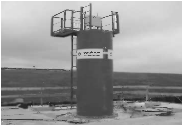
Figure 14.11 Typical tunnel access shaft. (Photo courtesy of NRA/DirectRoute.)
