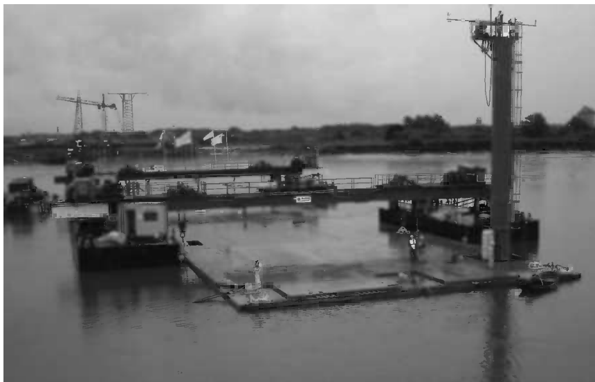
Figure 14.21 Limerick Tunnel immersion pontoons. (Photo courtesy of NRA/DirectRoute.)
