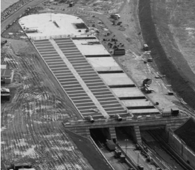
Figure 7.5 Øresund Tunnel portal with sunscreen (left) and rail pressure relief (right). (Photo courtesy of Øresundsbron.)
