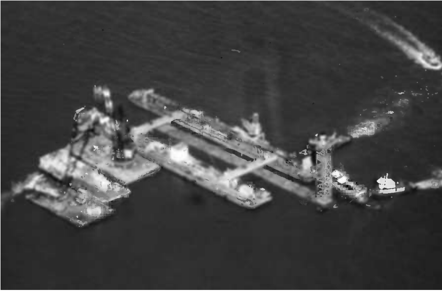
Figure 14.22 Lay barge on the Hampton Roads Tunnel. (Photo courtesy of W. Grantz.)
