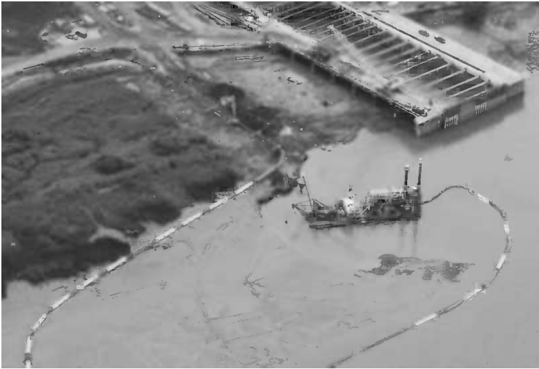
Figure 13.2 Cutter suction dredger on Limerick Tunnel. (Photo courtesy of NRA/DirectRoute.)
