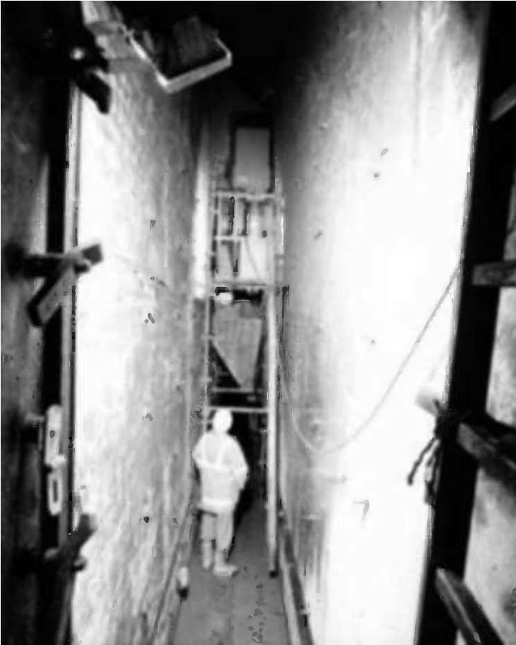
Figure 15.2 Bulkhead compartment. (Courtesy of Kent County Council, BAM Nuttall/Carillion/Philip Lane.)
