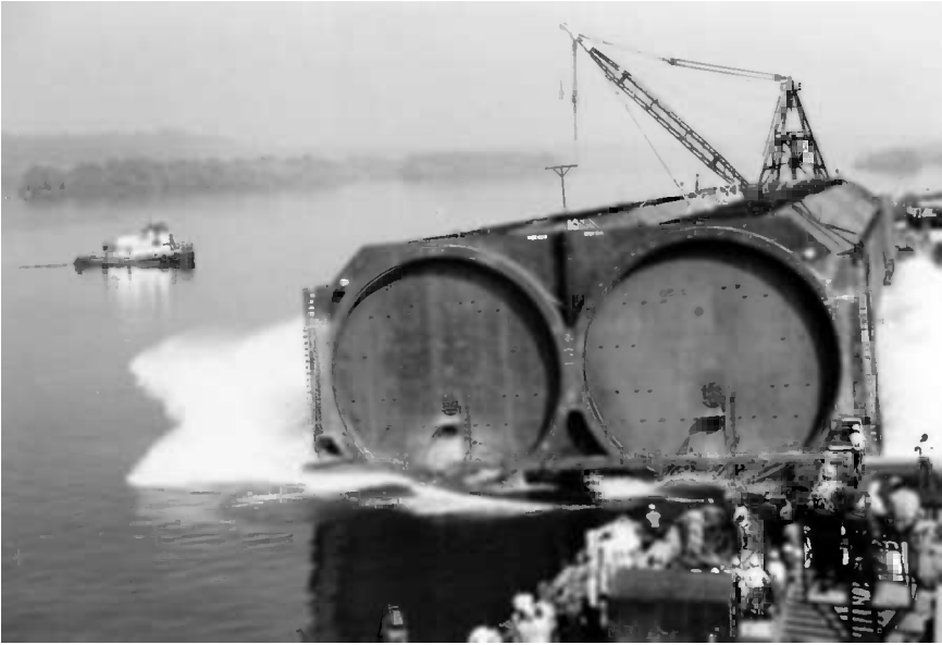
Figure 14.5 Launching a Fort McHenry Tunnel element. (Photo courtesy of W. Grantz.)
