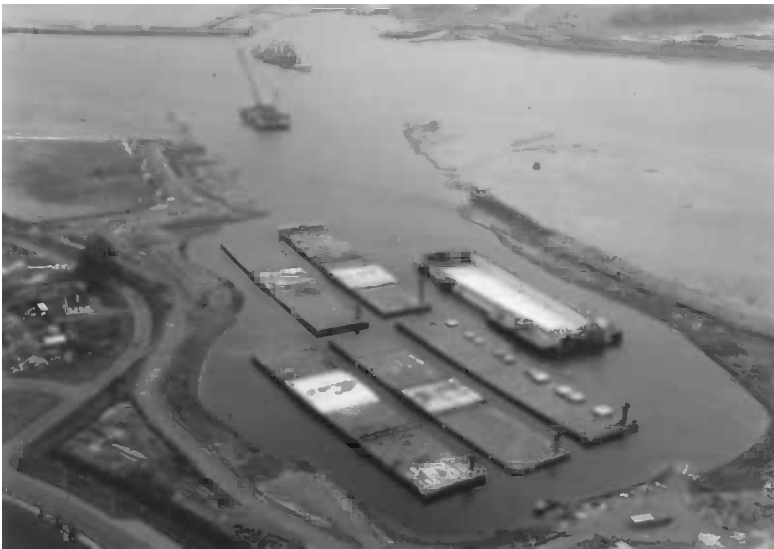
Figure 13.9 Jack Lynch Tunnel casting basin. (Photo courtesy of Cork City Council/Robert Bateman.)
