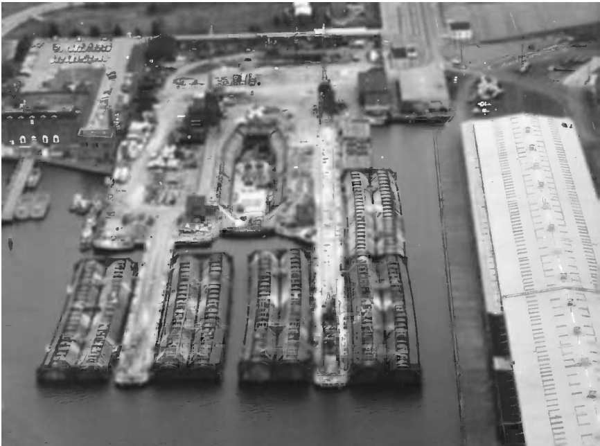
Figure 14.6 Concreting Fort McHenry Tunnel elements. (Photo courtesy of W. Grantz.)
