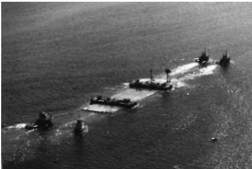
Figure 14.23 Concrete element being towed to site. (Photo courtesy of Øresundsbron.)
