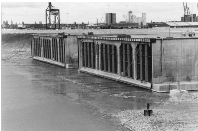
Figure 14.10 Demountable steel bulkheads. (Photo courtesy of Øresundsbron.)
