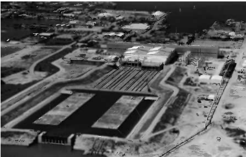
Figure 14.2 Øresund Tunnel casting facility. (Photo courtesy of Øresundsbron.)
