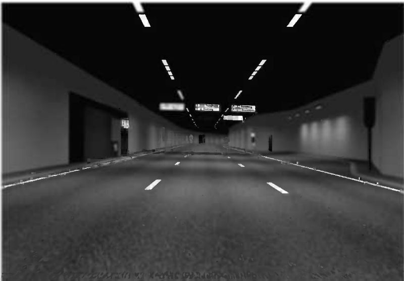
Figure 4.3 Plan and impression of lay-by in tunnel element. (Photo courtesy of Statens Vegvesen.)
