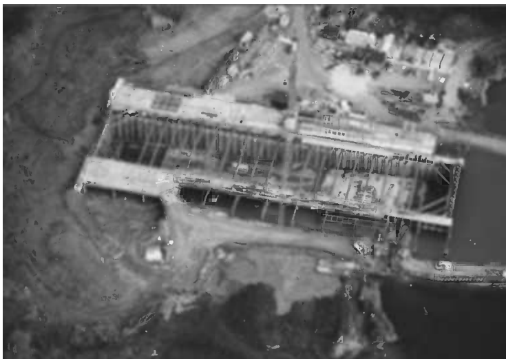
Figure 13.8 Limerick Tunnel cut-and-cover construction. (Photo courtesy of NRA/DirectRoute.)
