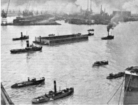
Figure 2.8 The Maastunnel under construction in 1941. (Photo courtesy of A. Scheel.)
