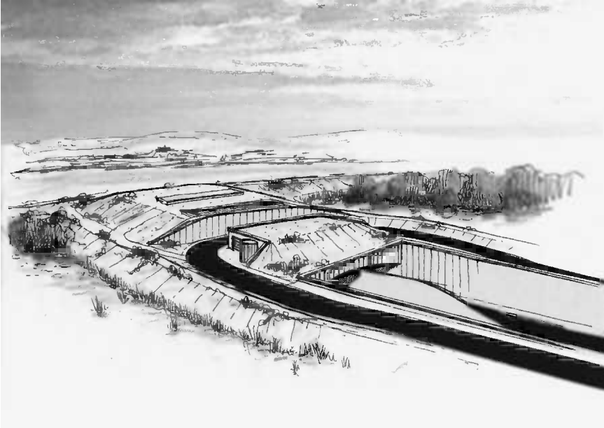
Figure 5.3 Limerick Tunnel service building within flood protection earthworks. (Courtesy of DirectRoute.)
