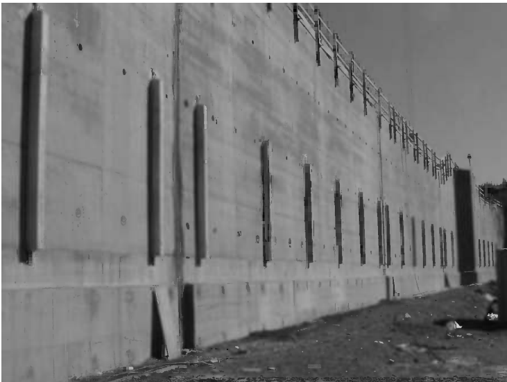
Figure 11.5 SACP anodes mounted on the exterior of the Bjørvika Tunnel.
