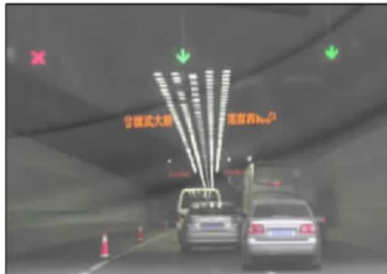
**Figure 13 The variable information board in tunnel**
