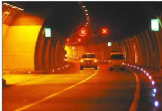
**Figure 12 Effective vision inducing facilities in tunnel**
