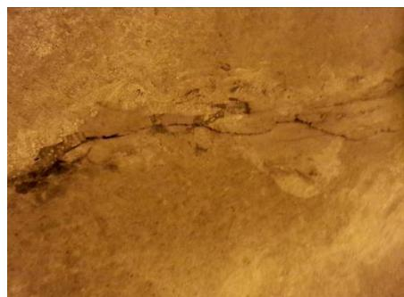
**Fig 1. Longitudinal crack of secondary lining**
