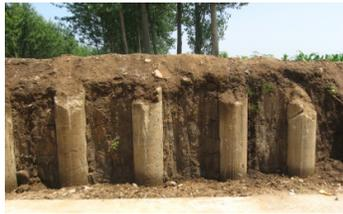
**Figure 4. CFG pile reinforced soft subsoil embankment**
