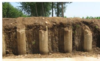
**Figure 4. CFG pile reinforced soft subsoil embankment**
