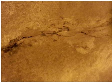
**Fig 1. Longitudinal crack of secondary lining**
