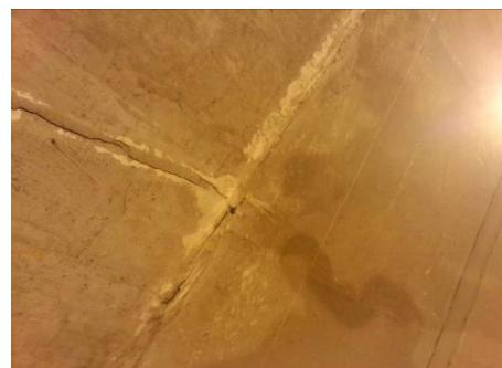
**Fig 2. Cross cracks of secondary lining**
