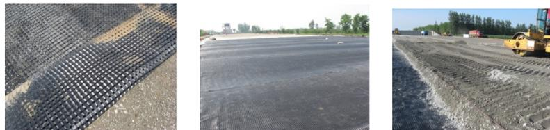
**Figure 5. In the Cement Grade Macadam filled with two layers horizontal geogrid reinforcement on top of the piles**
