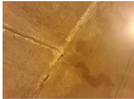
**Fig 2. Cross cracks of secondary lining**
