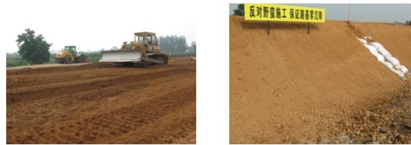
**Figure 6. Embankment fill**
