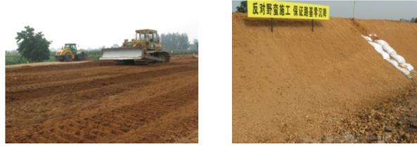
**Figure 6. Embankment fill**
