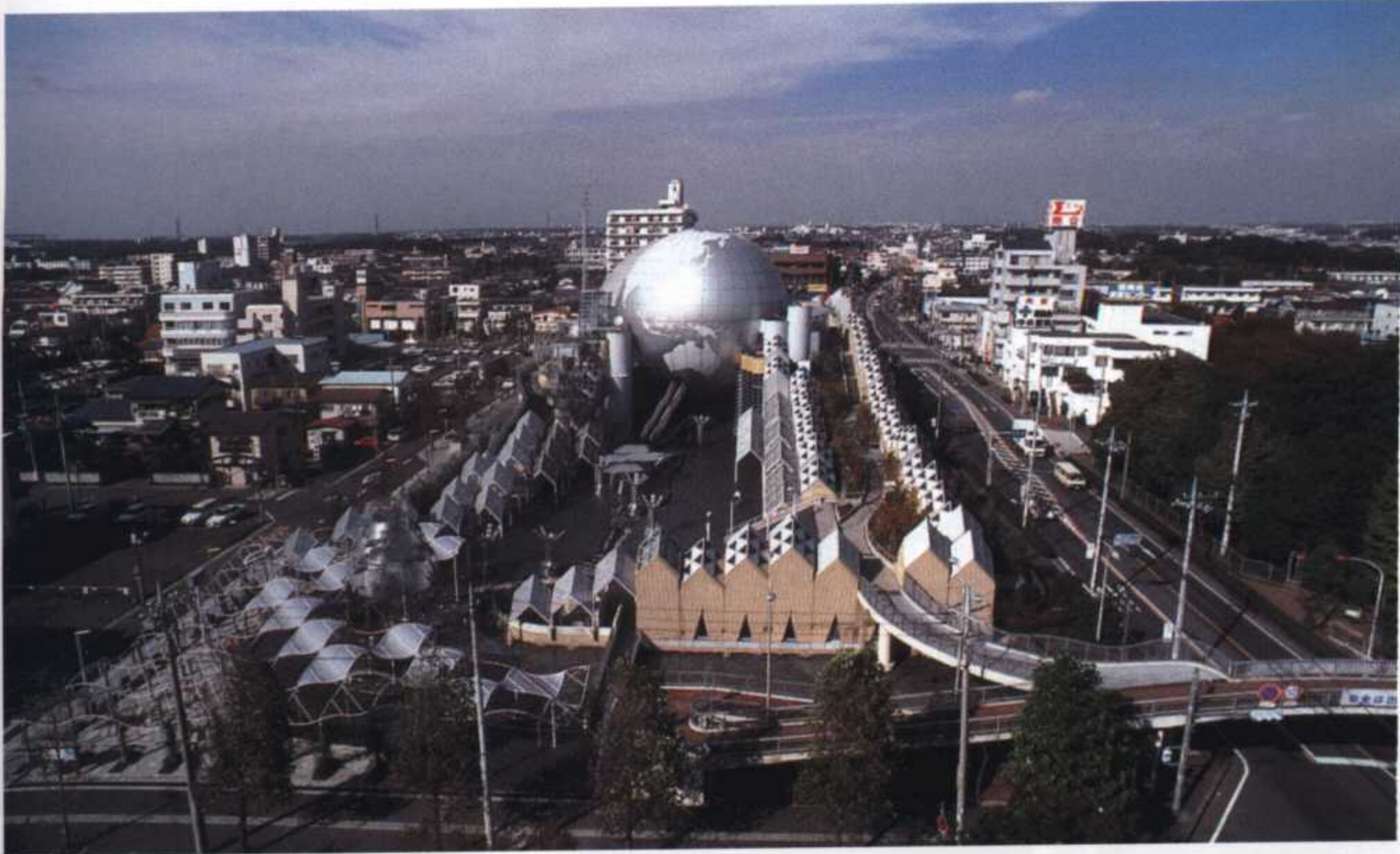
1 Site plan 2 Overall view from the south 3 Overall view from the southwest
