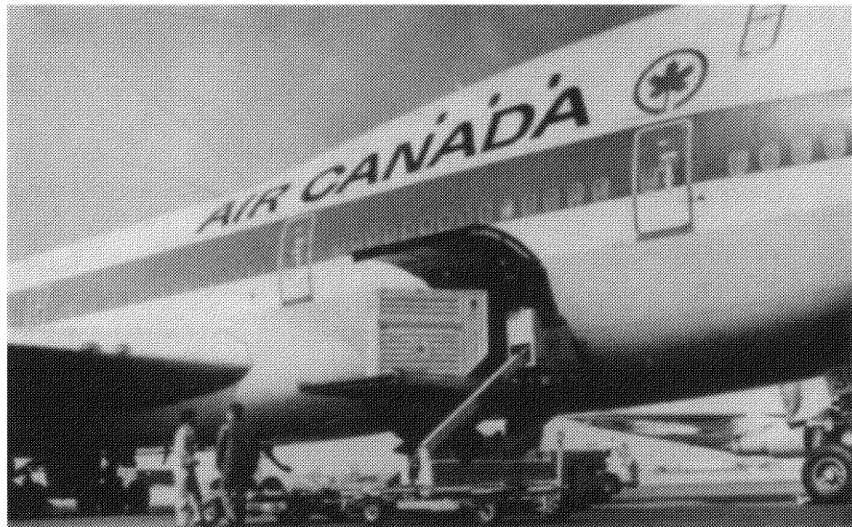
FIGURE 11.8 Palletized unit being transferred to an aircraft.
