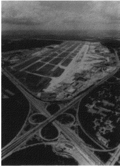
FIGURE 13.8(b) Land side access layout—LaGuardia Airport, New York). Courtesy: The Port Authority of New York and New Jersey.
