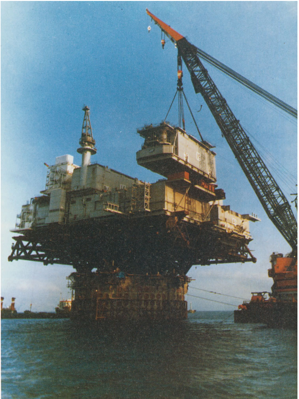
Fig. 24 : Installation of modules
