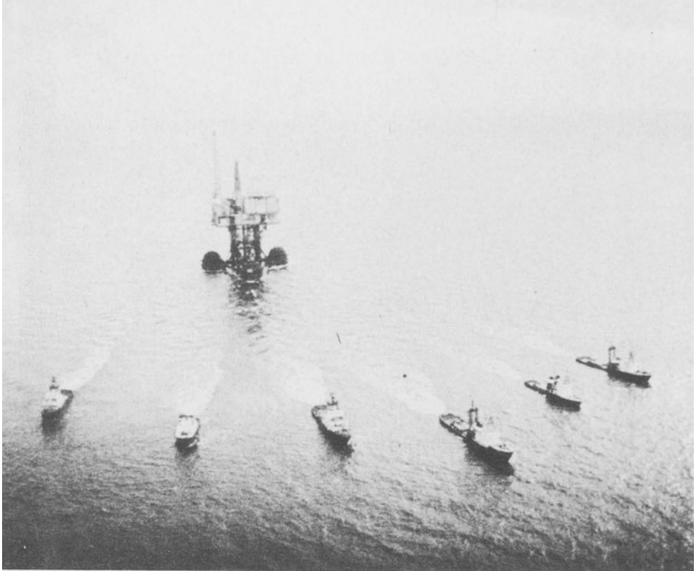
Figure 21 - Platform during Second Tow
