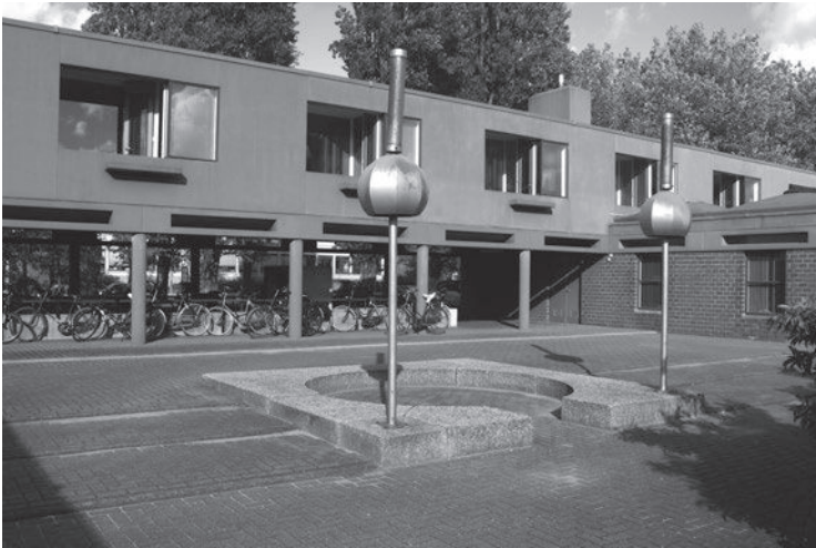
‘Counter-practices’, Amsterdam Orphanage, Amstelveenseweg, Amsterdam (1955–1960), Aldo van Eyck, Architect
