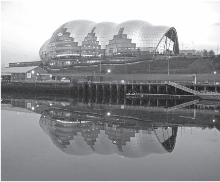
Sage Gateshead, Gateshead, UK, Foster + Partners, Architects (1997–2004)
