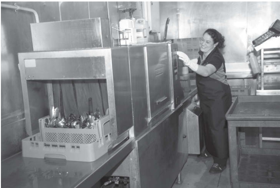
Figure 4.5 Automated dish machine; circular design.
