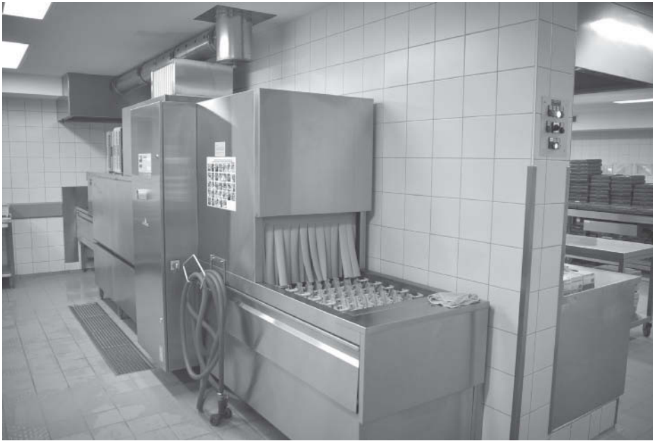
Figure 4.4 Double-tank automated dish machine.
