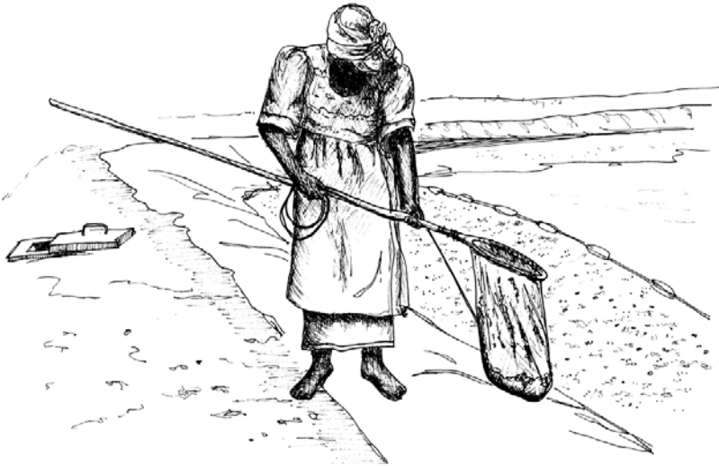
Figure 22-4. Surface Plants, Scum, and Unwanted Algae Can Be Removed by Manual Cleaning with a Rake, Skimmer, or Net.
