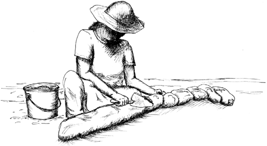
Figure 7-25. A Masonry Rock Wall Being Constructed as a Wash Area Wall. To Save Purchased Materials, Rocks Are Placed in a Bed of Mortar and Then Covered with Mortar.
