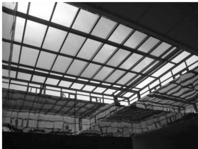
Figure 4. Prismatic glazing on the atrium (Kushan Hushi electronics office building).
