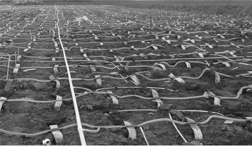
Figure 10. Assembly of pipeline system.
