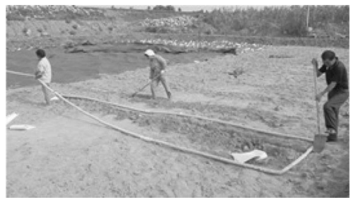
Figure 9. Construction of the sand layer.
