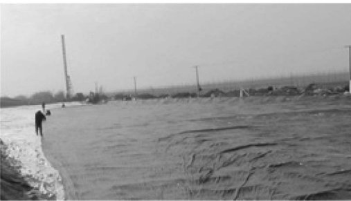
Figure 12. Laying of airtight HDPE membrane.
