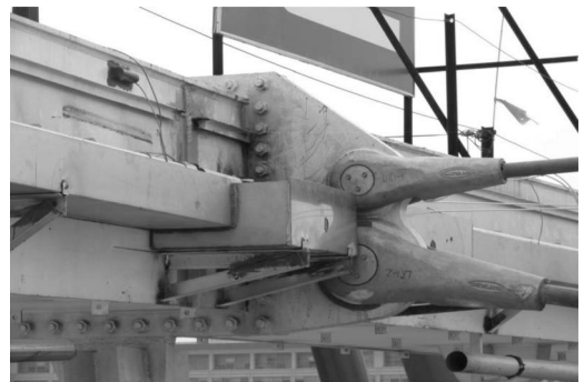
Figure 2. Unadjustable anchor end of cable.
