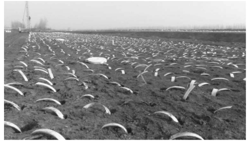
Figure 8. Installation of PVDs.
