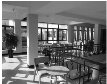
Figure 5. Combined prismatic and conventional glazing (Shanghai green building technology incubator building).
