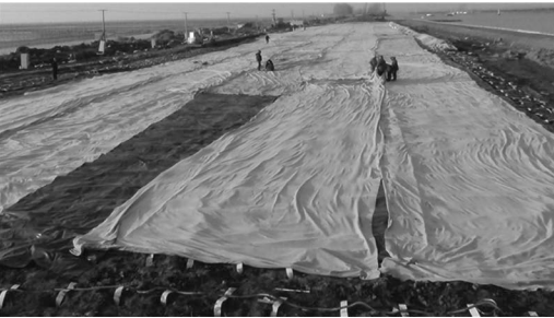
Figure 11. Laying of protection geotextile.
