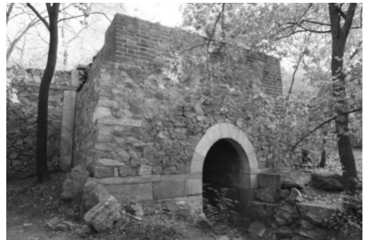
Figure 7. Difference between the repair material and original architectural material for Clock Pavilion.
