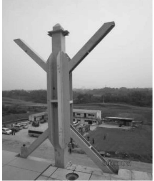
Figure 4. Diagonal braces column.
