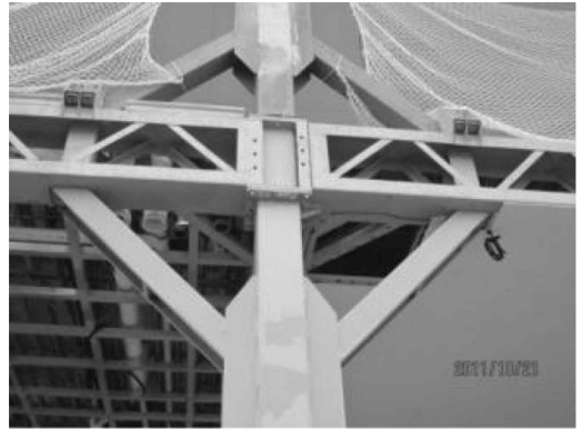
Figure 5. Diagonal braces joint.
