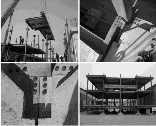
Figure 1. Assembly experiment of two-floor structure.
