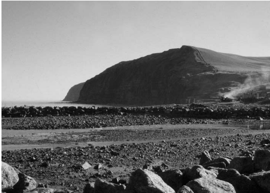
Looking south, fishtail groyne in centre ground
