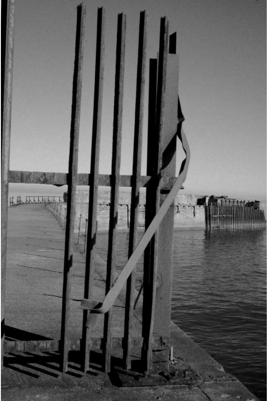
A gap in the fence
