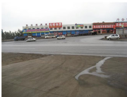
Before improvement of national highway G307
