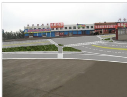
After improvement of national highway G307
