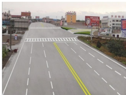
After improvement of provincial highway S340
