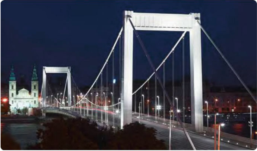
Fig. 9 Ceramic metal halide lamps in streetlighting. Image from GE Lighting
