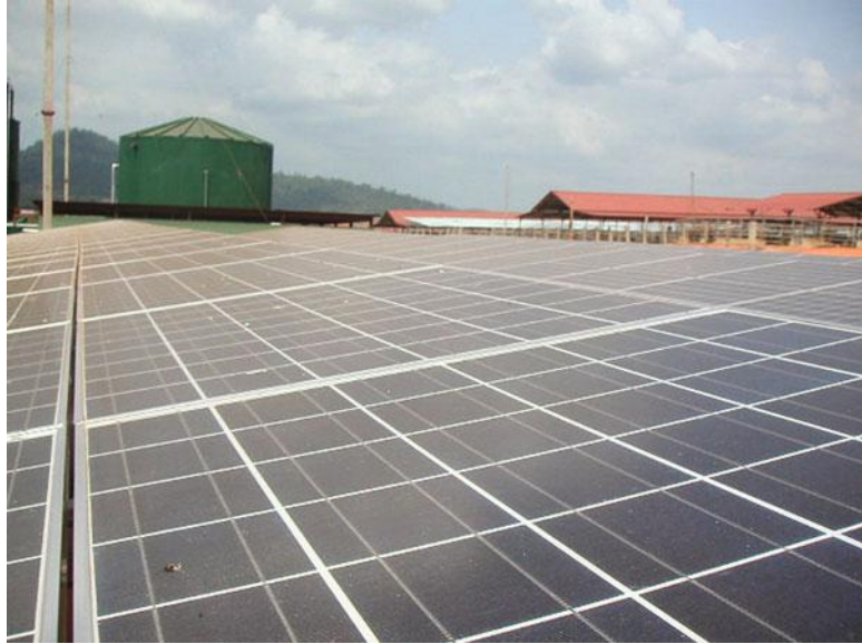
Figure 12.1 Dusty modules will have a reduced yield
