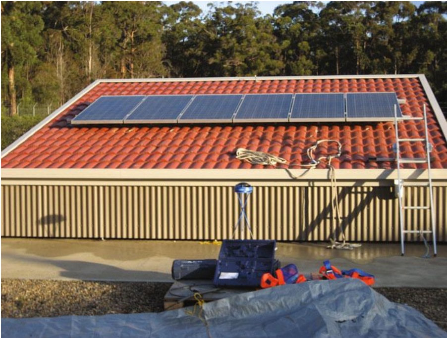
Figure 7.6 Solar Pathfinder in use
