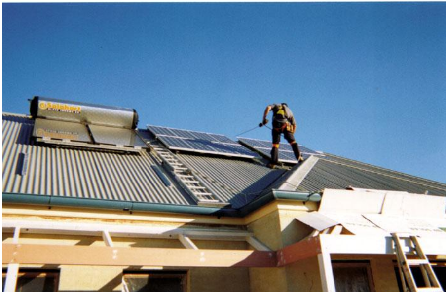
Figure 1.3 An electrician installing a solar system that includes both a solar hot water system (left) and a solar electric system (right)
