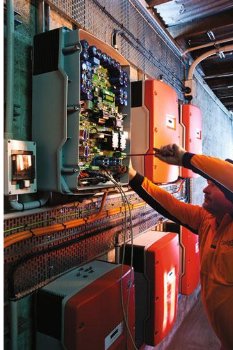
Figure 5.12 Multi-string inverters installed by Solgen Energy on Cockatoo Island for Sydney Harbour Federation Trust
