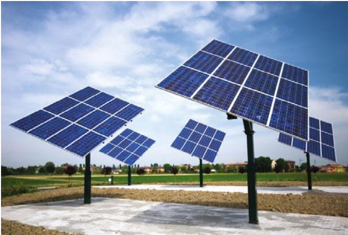
Figure 6.16 Sun-tracking system: the arrays rotate throughout the day to face the sun
