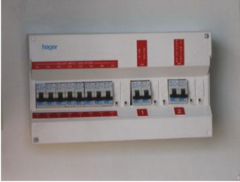
Figure 5.26 Circuit breakers in a grid-tied PV system
