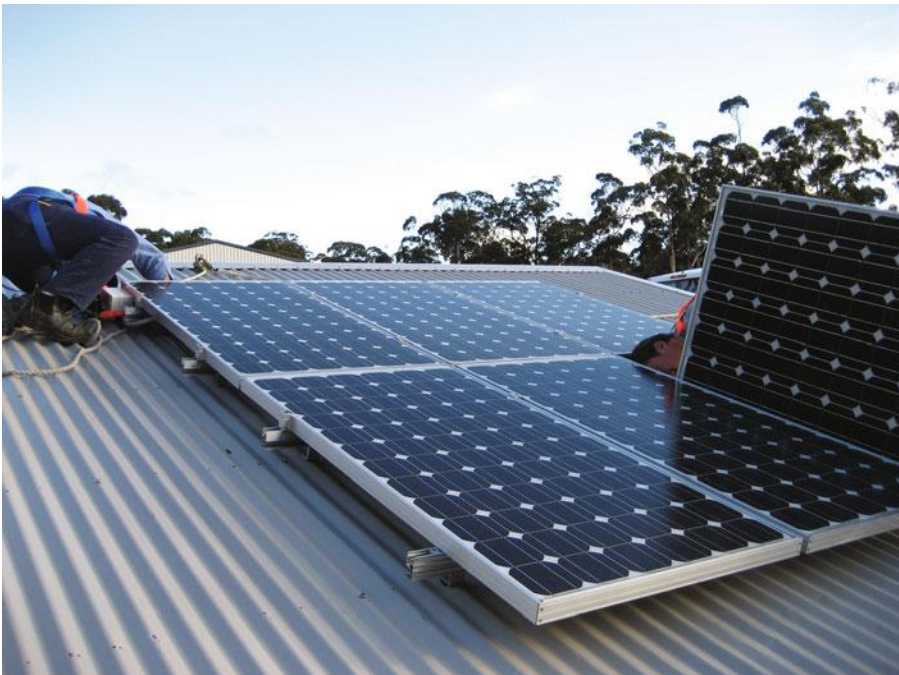
Figure 6.6 Corrugated metal roof installation
