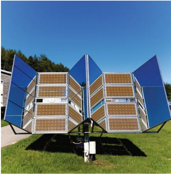
Figure 3.14 The mirrors either side of the module are used to concentrate light and increase power output
