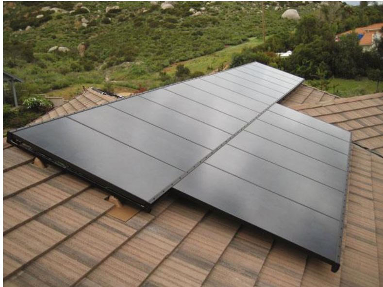
Figure 14.23 The mounting system achieves a good balance between aesthetics and performance. It is elevated slightly above the roof to allow for cooling ventilation but still retains a low profile and blends in with the roof face
