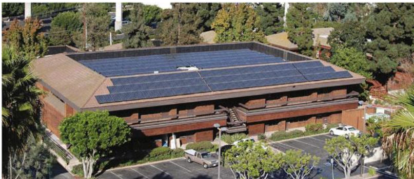
Figure 14.11 The greatest design challenge for this installation site was the limited available roof space. To overcome this the designer mounted modules facing south on the tile roof in addition to modules tilted south on the flat roof
