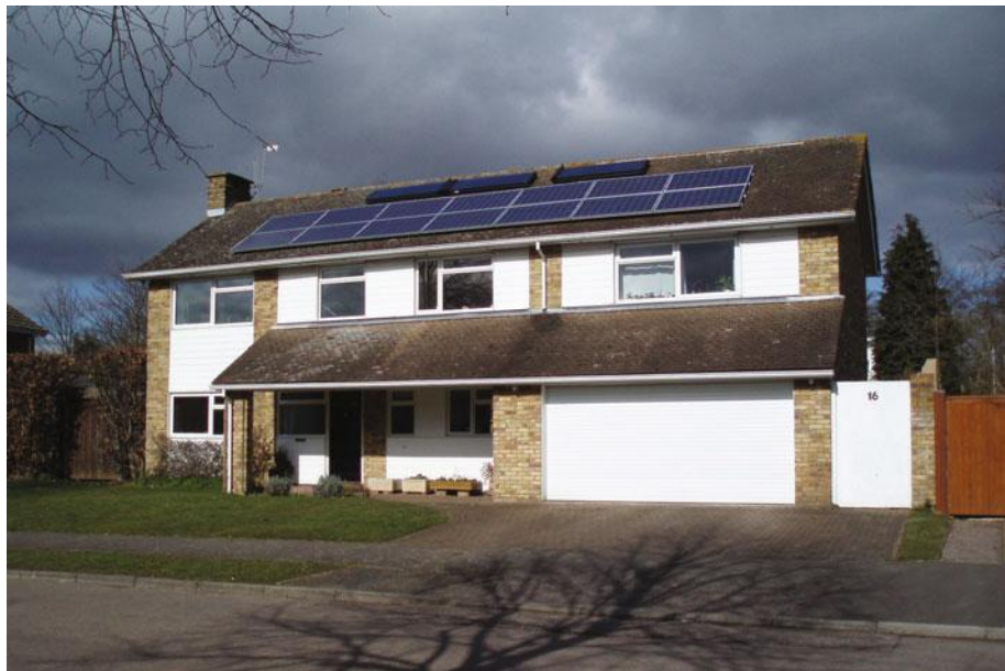
Figure 14.9 In order to meet the household energy demands 14 PV modules and 3 solar thermal collectors have been installed
