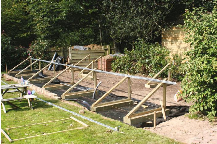
Figure 14.34 Construction of the mounting structure, the wooden A-frames and Unistrut strip (along the top) can be seen. Another strip of Unistrut can be seen on the grass; it will be attached along the bottom of the A-frames
