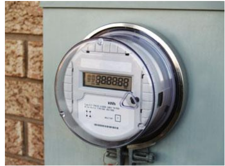
Figure 5.35 A more complex digital meter also known as a smart meter; many governments and utilities have started to introduce smart meters, which are expected to be very widely used in future
