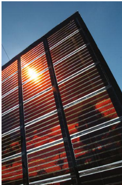
Figure 3.10 Dye solar cells are available in a range of attractive colours and are transparent so they can be integrated into the facade of a building
