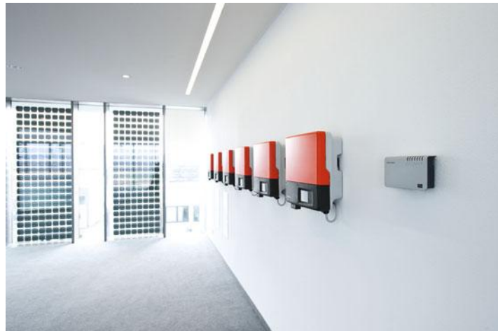
Figure 5.4 A transformer-less inverter is generally smaller, lighter and more efficient than an inverter of the same size (in kW) with a transformer
