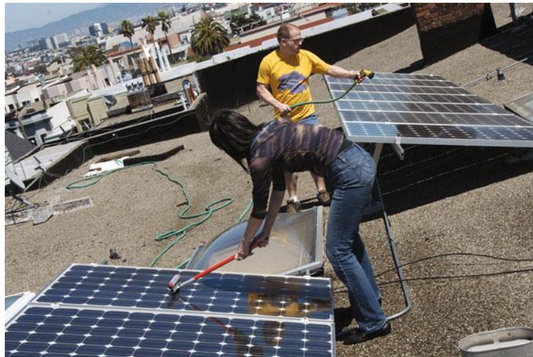
Figure 12.2 Cleaning a PV module involves spraying them with a hose and occasionally scrubbing to remove baked-on marks
