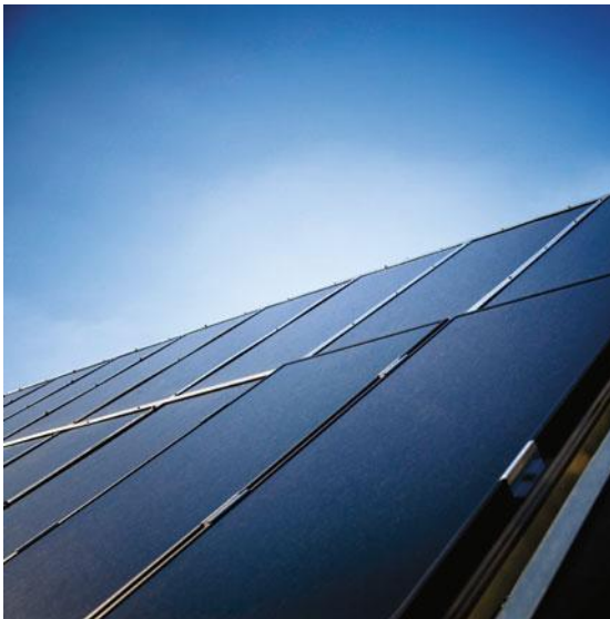
Figure 3.5 Amorphous silicon modules are easily distinguished from crystalline modules by their dark and uniform colour but they also look like non-silicone thin film modules
