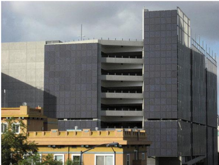
Figure 1.10 A 40kWp commercial grid-connected PV system located in San Diego, California. The modules have been mounted vertically because the roof space is used as a car park
