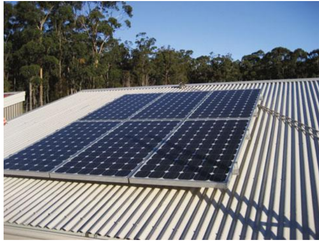
Figure 4.22 Even this small shadow can reduce the amount of electricity a module produces – a small shaded area can, under certain circumstances reduce module output by 80–90 per cent as well as affecting the rest of the array
