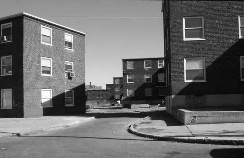
Figure 4.13 Orchard Park, Boston (1993). This public housing project, completed in 1942 as a maze of three-story walk-up buildings, suffered from serious deterioration after 50 years of occupancy and inadequate maintenance. (Source: Lawrence Vale)
