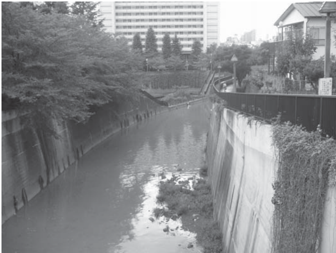
Fig. 3.15 Large capacity of an urban river channel
