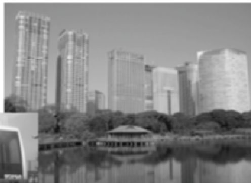
Office building district using reclaimed water for toilet flushing
