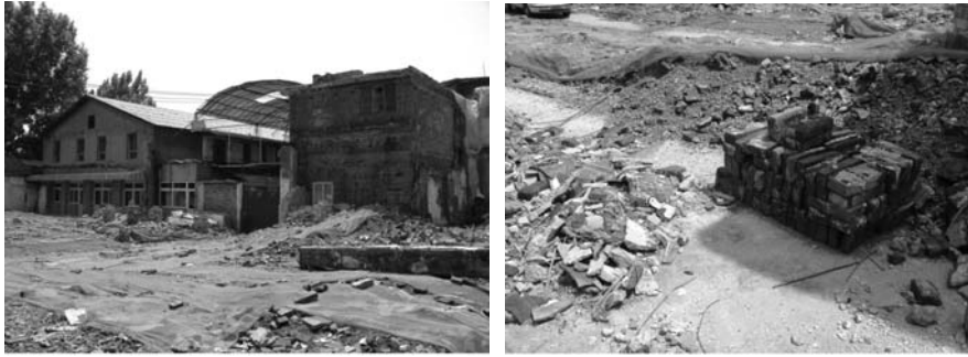
Fig. 6.25 Dismantlement site in Beijing
