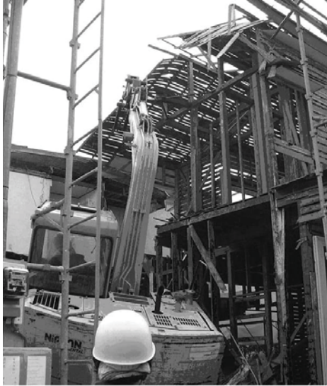
Fig. 6.16 Dismantlement by machine
