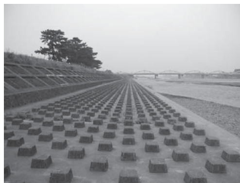
Fig. 3.6 Projections to increase the roughness of the surface
