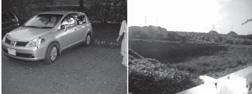
Fig. 3.20 Countermeasures to retain water in a drainage basin: permeable pavement in a parking area (left) and a retarding basin (right)
