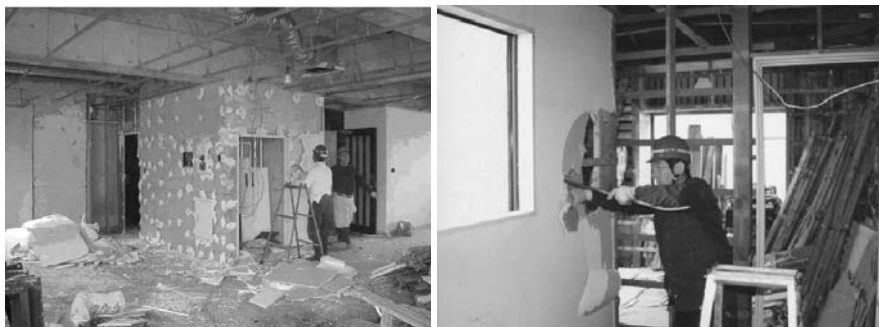
Fig. 6.14 Interior finishing removal process
