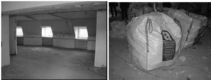
Fig.6.17 The separation of the inner wall and separation of the asbestos
