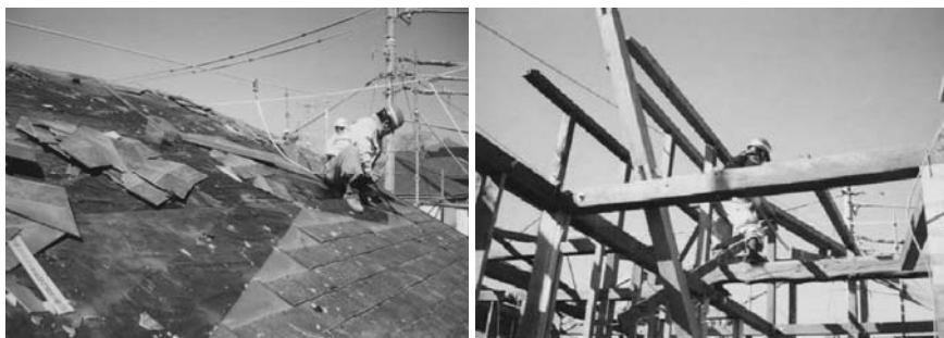
Fig. 6.15 Dismantlement by hand
