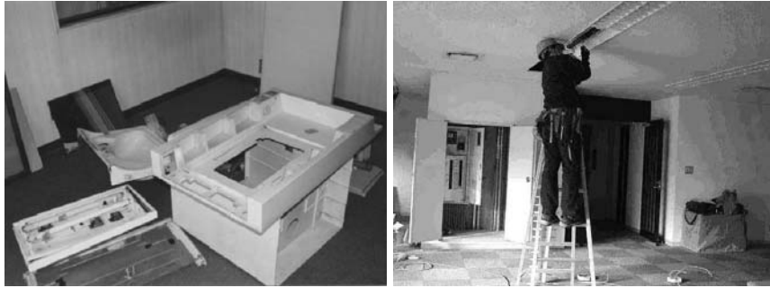
Fig. 6.13 Equipment removal process
