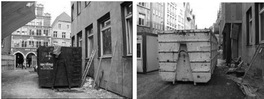
Fig. 6.19 Container for collecting material wastes
