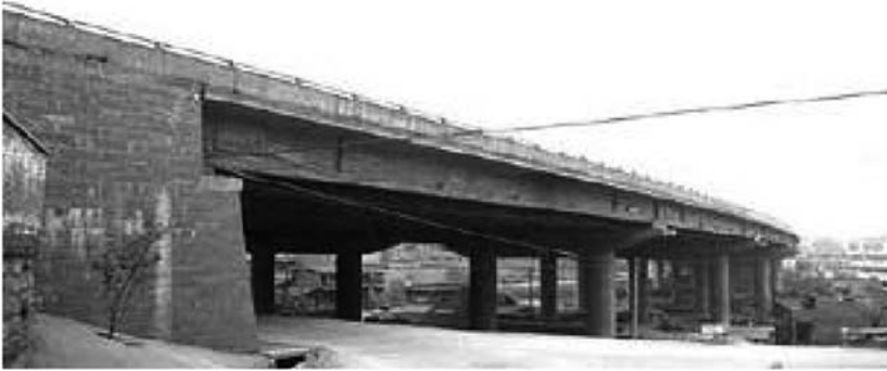
Figure 6.2 Photograph of the Hongcaofang Crossroads Bridge.
