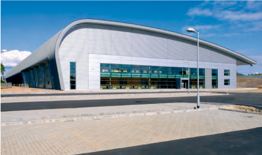
Figure 5.19 Curved steel sections used in a modern industrial building in the UK
