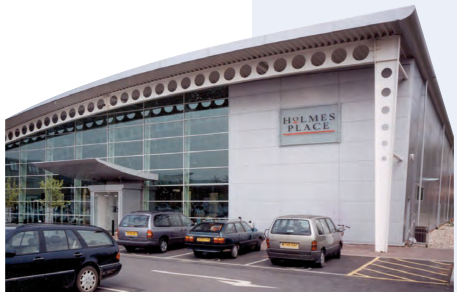
Figure 1.1 Leisure building using a steel framed structure
