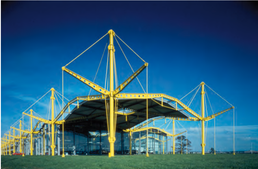
Figure 2.14 Suspended structure used at the Renault Factory, Swindon, UK built in the 1980's Architect: Richard Rogers Partnership
