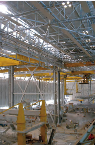
Internal view of the building during construction
