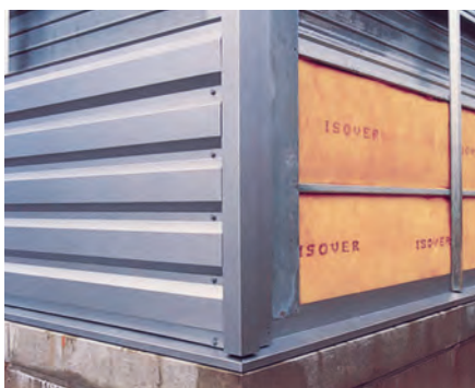
Figure 5.5 Trapezoidal roll-formed profiled sheet fixed to liner trays
