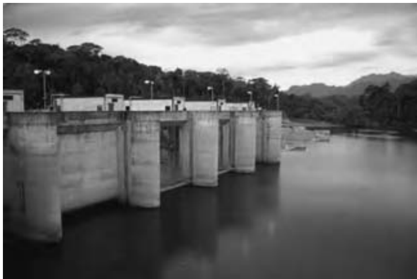
Figure 9.3 Theun-Hinboun Dam wall
