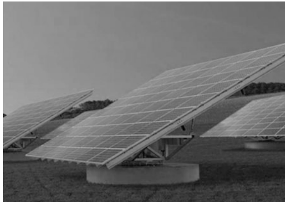
Fig. 7.6 Azimuth one axis tracking system
