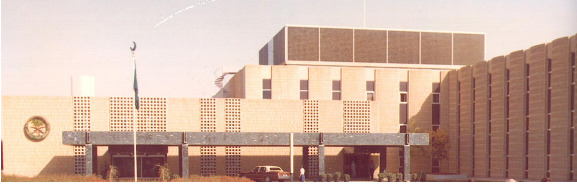
The King Faisal Hospital and Research Center, Riyadh, Saudi Arabia
