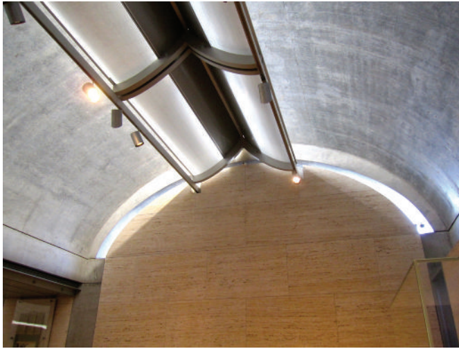
Figure 14: The Kimbell Art Museum, detail of the clear-span cycloid concrete shell, Louis Kahn.
