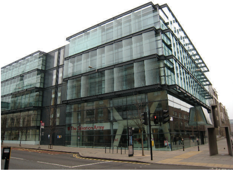
Figure 41: Façade clad with laser cut panels, London.
