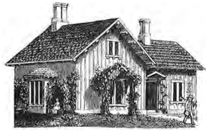
cottage with bracketed eaves
