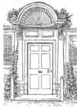
bracketed hood above a door
