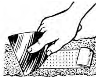
perforated tape covering a joint
