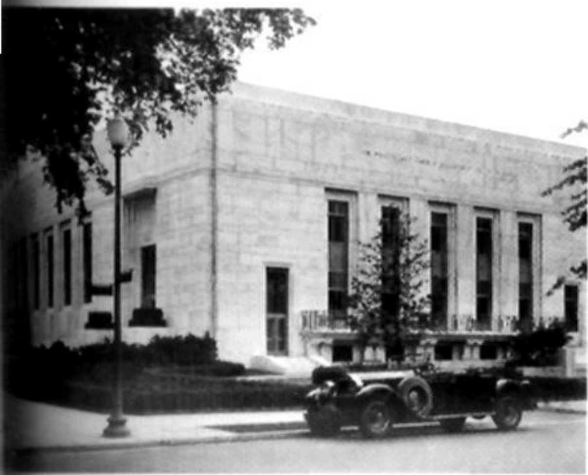
Paul Philippe Cret's Folger Shakespeare Library in Washington, D.C., was a sober stone pile of 1932, designed in collaboration with Alexander B. Trowbridge. Often referred to as 'Greco Deco', the clean-lined, classically proportioned pile nonetheless included strong modern statements in its abundant use of cast aluminium (for windows, grilles and railings) and its novel ground-level placement of nine bas-relief panels depicting scenes from Shakespearian plays.
