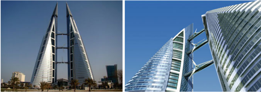
Fig. 3 Bahrain world trade centre-installation of wind turbines on the building. Source Internet
