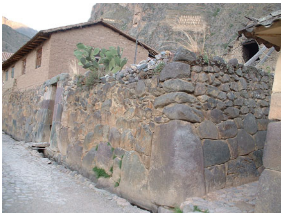
Fig. 1 External view of a kancha wall at Ollantaytambo, Cuzco. Note the wall camber, sturdy corner blocks and trapezoidal doorway (Photo: Mackay 2007)
