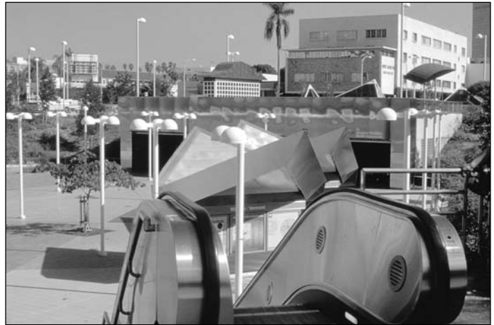
Access plaza to the Los Angeles Red Line.
