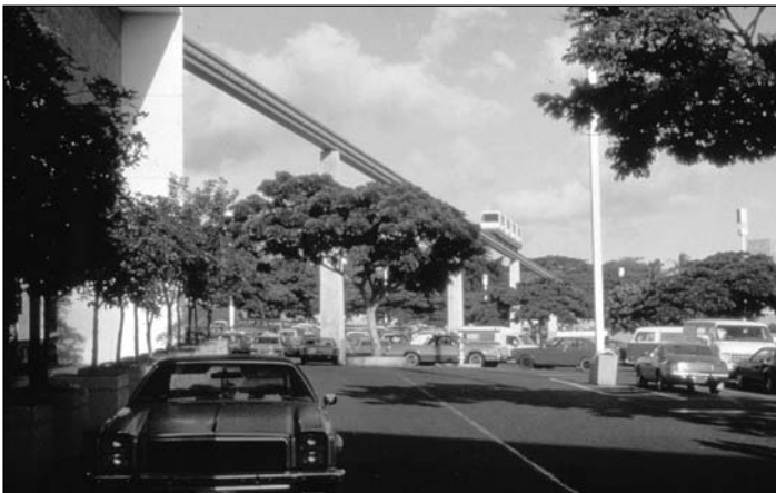
Service to commercial development in Honolulu.
