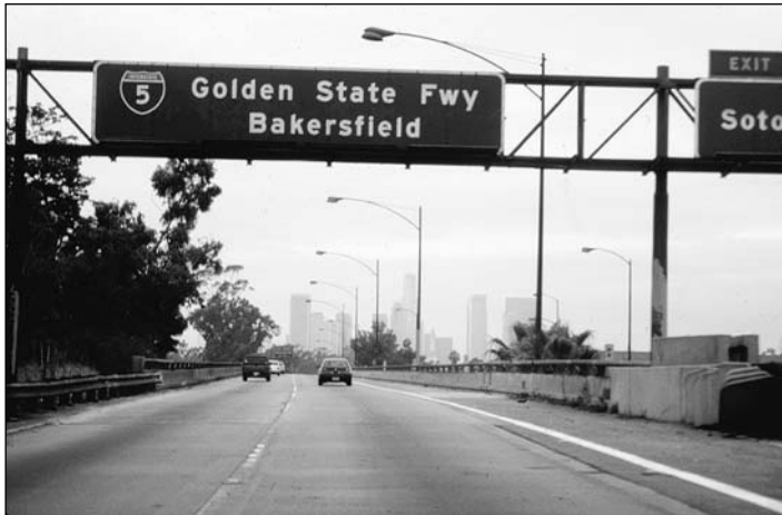
Typical urban highway view, with the skyline ahead (Los Angeles).
