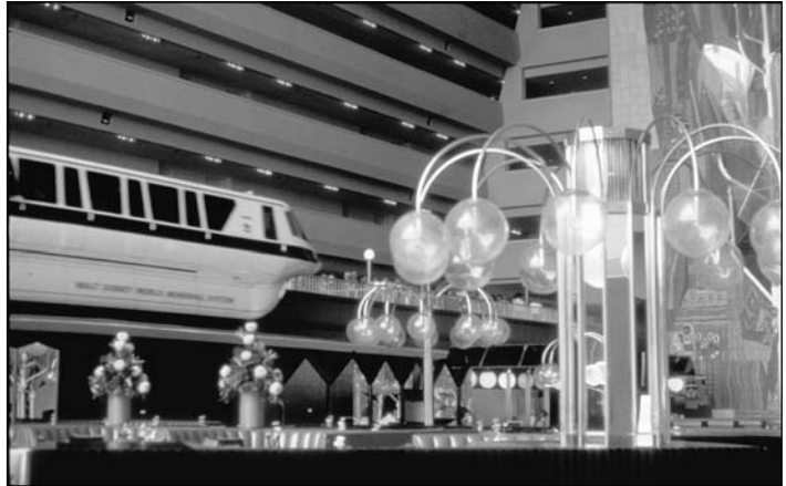
Service line penetrating the atrium of a Disney hotel.
