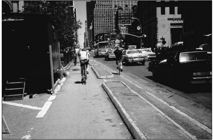
Segregated bike lane with barriers on Sixth Avenue in New York City.
