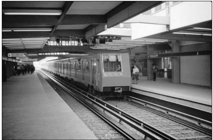
Mexico City metro operations, utilizing cars with rubber tires.
