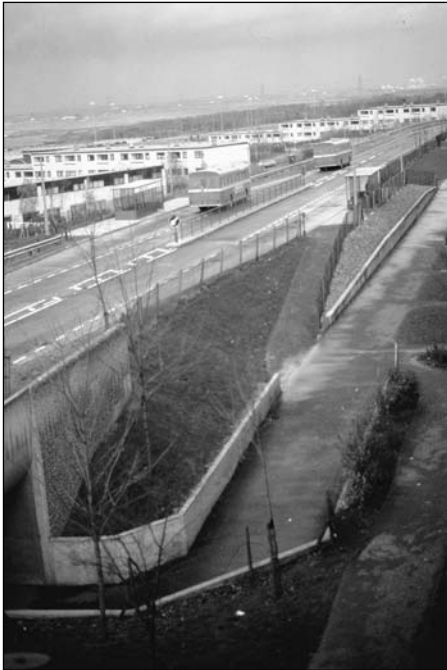
Busway with pedestrian underpass in the British new town of Runcorn.
