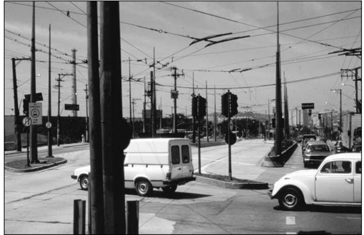
Overhead power lines at a trolley depot in São Paulo.
