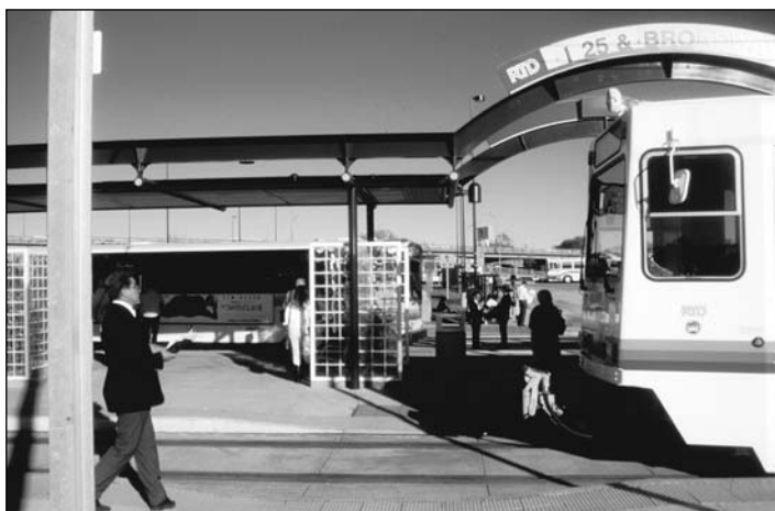
Low-platform station in the Denver LRT system.
