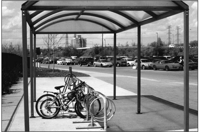
Bicycle parking at a station of the Ottawa busway.
