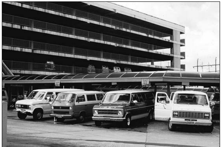
Paratransit (Caguas) terminal and garage in Puerto Rico (Bayamon).
