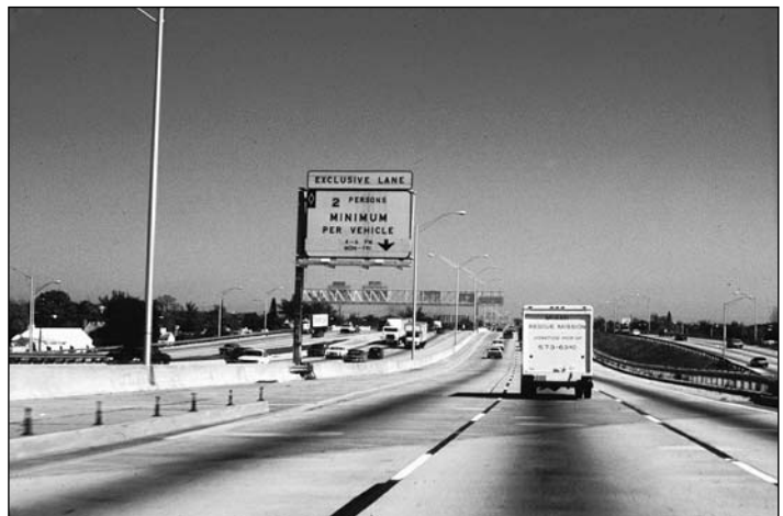
Highway in Miami with signs pointing to HOV lanes.
