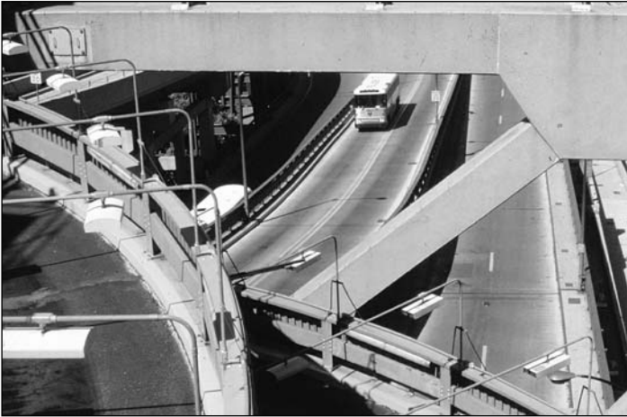
Access ramps from the rear of the Port Authority Bus Terminal in New York City.
