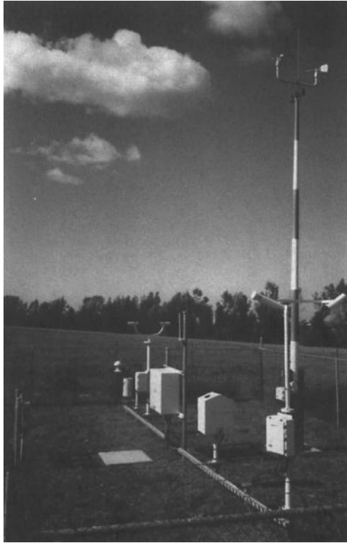
FIGURE 82.6 A view of an ASOS system sited at an airport near San Diego. The instrument of Figure 82.5 is seen in the foreground. A stand for the freezing rain sensor is not used. The next instrument is the ceilometer. Behind that is a metal box containing connections to the sensors and instruments to transmit the data to a remote collection and processing station. Along the same line of instruments beyond this is the precipitation identification or present weather sensor. This is followed along the same line by the sensor measuring ambient and dew-point temperatures and a tipping-bucket rain gage. To the north of the line of instruments is a pole with a cup anemometer, weather vane, flashing red lights, and lightning rod at the top.
