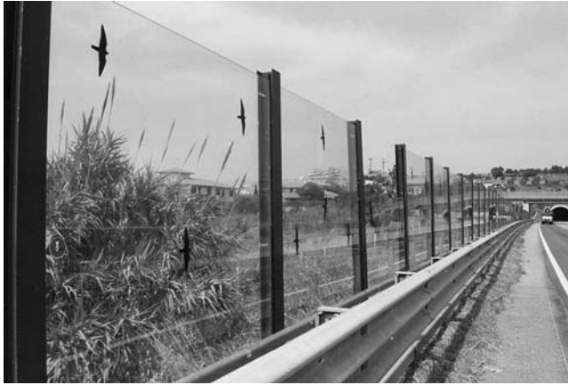
Figure 24.2 Transparent noise barriers along a national road (San Vincenzo, in province of Livorno). Attached on them are silhouettes to prevent collision with birds (M. Dinetti, 1997).
