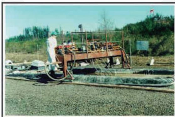
40 Cubic Yard Demonstration
