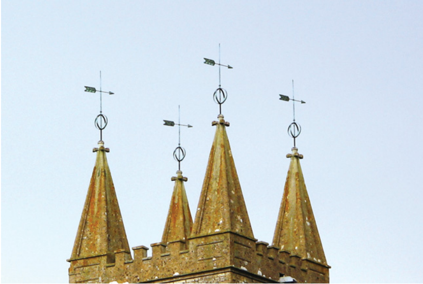
Figure 8.8 Ornate weather vanes receive varying amounts of maintenance, and are unlikely to have low friction bearings. A combination of several devices provides more confidence in the direction indicated.
