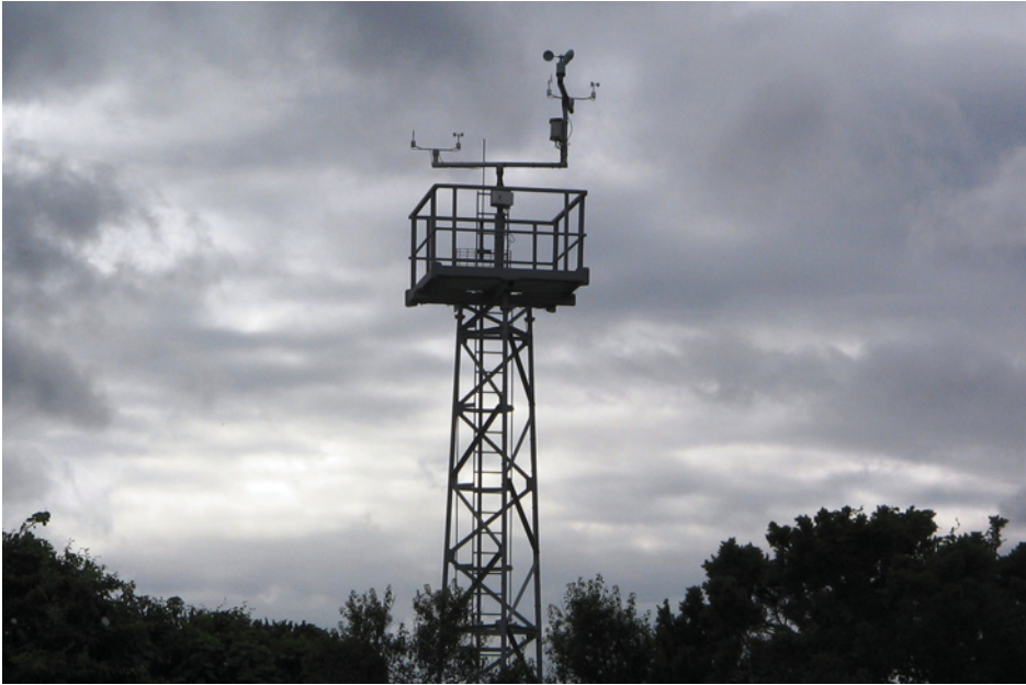
Figure 8.12 Standard meteorological mast at Camborne Met Office, Kehelland, Cornwall, carrying anemometers and wind vanes.
