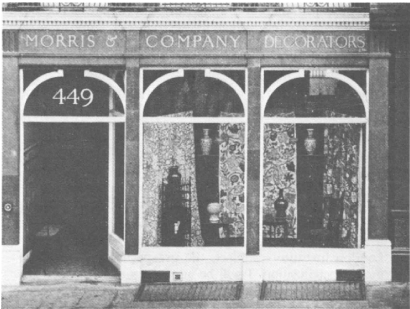
3.2 Morris & Company showroom, 449 Oxford Street
