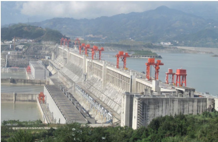
Fig. 5.5 Photograph of the HPP Three Gorges (China)
