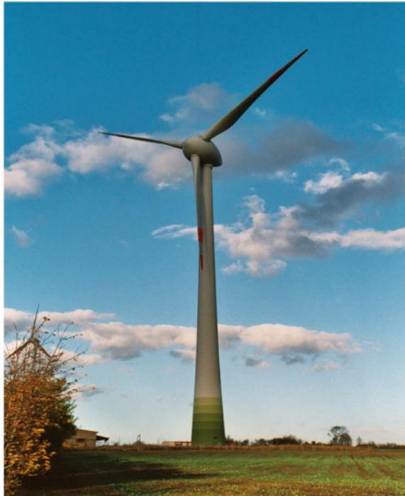
Fig. 5.8 Photo of a 4.5 MW windPP with a diameter of 112.8 m and a gondola at a height of 180 m above the ground
