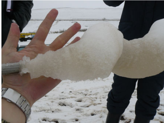
Fig. 6.5 Ice on the wire of OTL-110 kV
