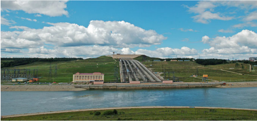
Fig. 7.5 Administrative building and water lines (penstocks) of Zagorskaya PSPP
