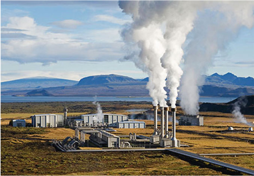
Fig. 5.24 Typical external view of the GTPP
