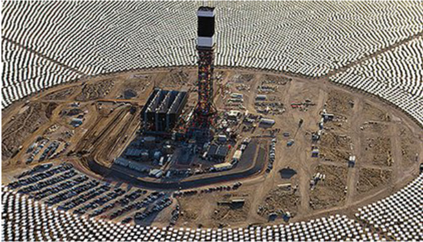
Fig. 5.13 Ivanpah Solar Electric Generating System (Desert Mochava, USA). Characteristics: power—392 MW, footprint on the Earth—13 km 2 , mirrors quantity—350 thousand, boilers at height of 140 m, cost—$2.2 billion
