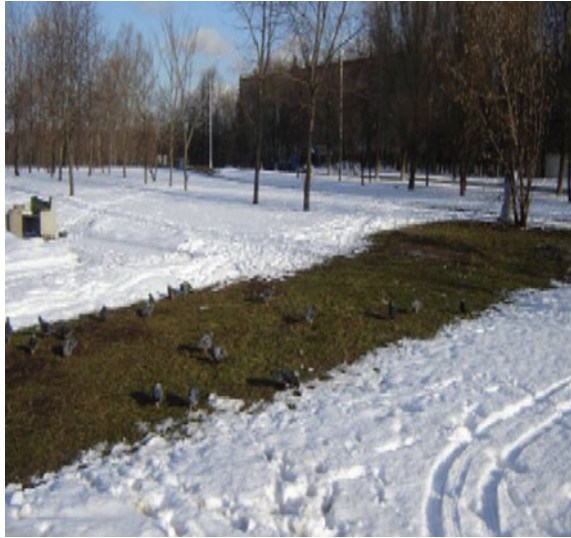
Fig. 8.12 Illustration of poor quality thermal insulation of pipes of transport systems of thermal energy
