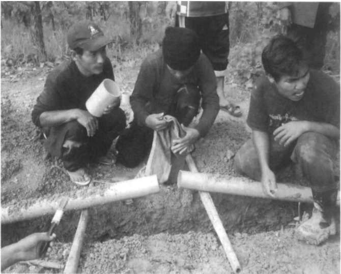
Figure 1.4 Workers preparing to glue a PVC pipe joint.
