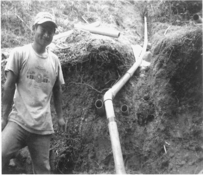
Figure 1.5 A 22.5° elbow joining PVC (top) and galvanized iron pipe (bottom).
