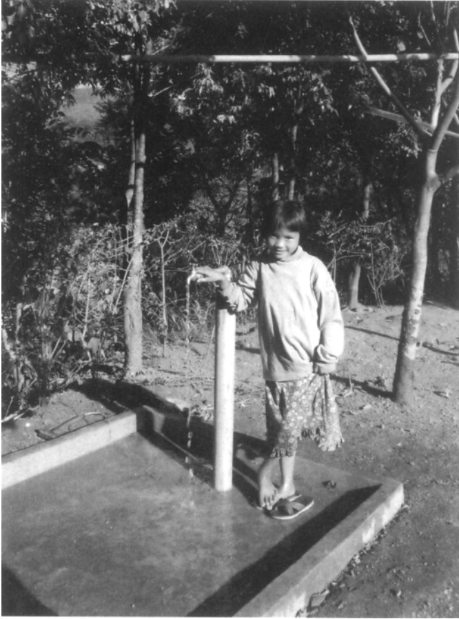
Figure 1.12 A completed tapstand.
