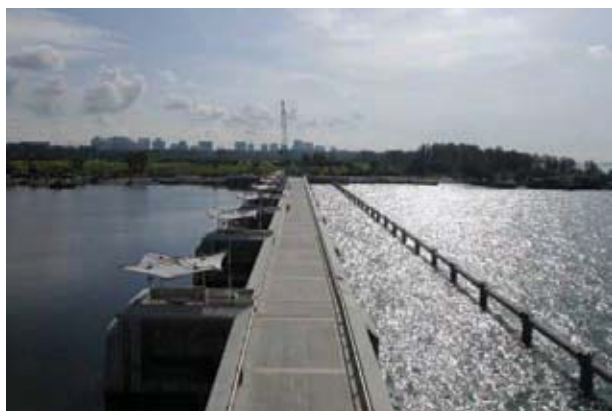
Figure 11 The Marina Barrage
