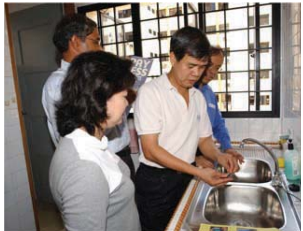
Water conservation: Installing water-saving devices in residents' homes in Singapore.
