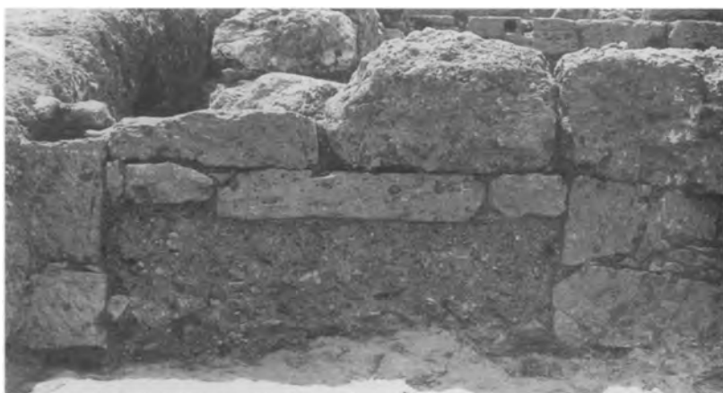
b. P:25, blocked entrance in Wall 2 (from north).
