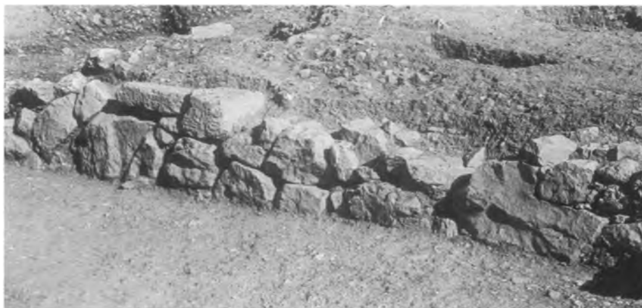
c. I-J:16-17, road retaining wall (from north).
