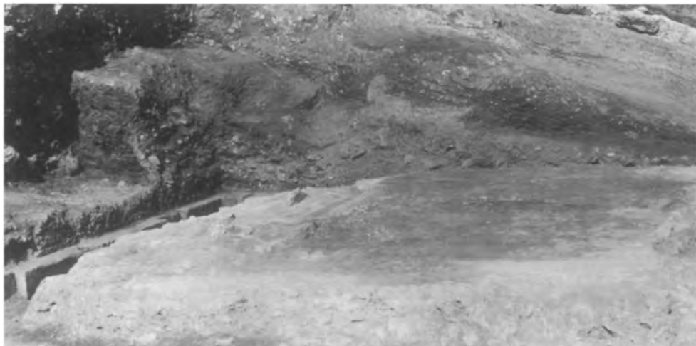
b. Construction packing behind walls of Building T-U:19 (from northeast).
