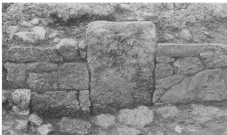
b. Building K-L:21-22, Room 1, south wall (from north).
