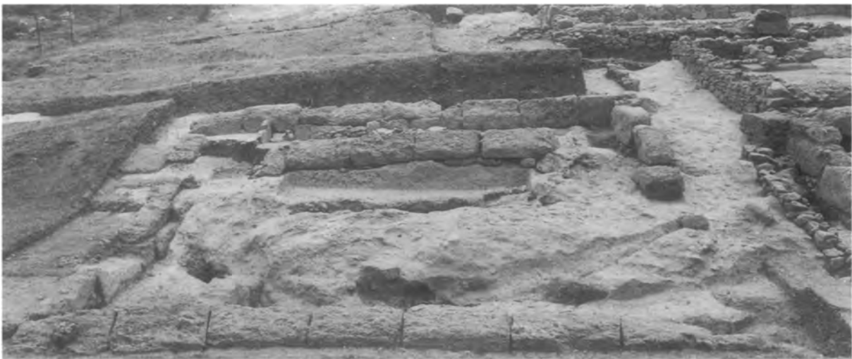
c. Building N:28 (from north).
