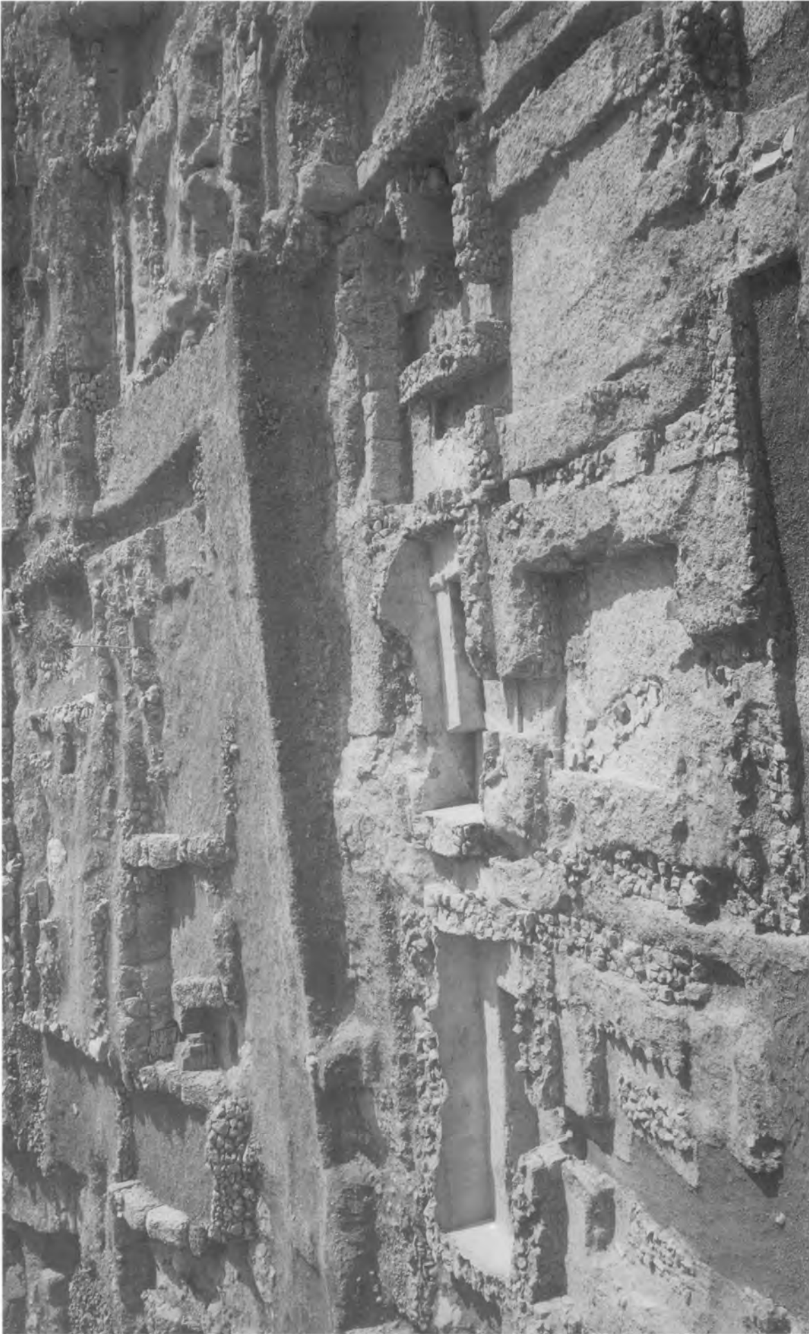
Left to right, Buildings L:26-27, K-L:25-26, K-L:24-25 (from north); to south, Building M-N:25-26 at left, M-N:20-24, Rooms 3 and 4 at right.
