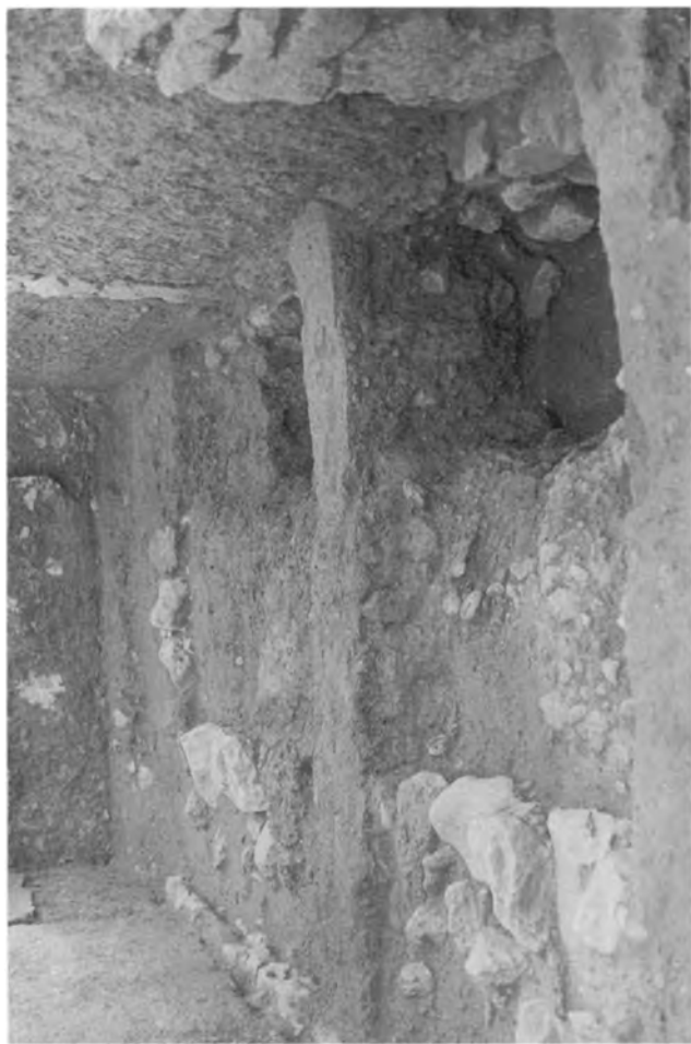
a. Building M:16-17, Room 2, test below floor; east wall of M:17-18 at left.
