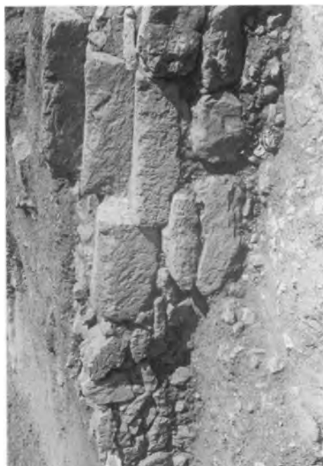
e. Secondary entrance in K:14 (from northwest).
