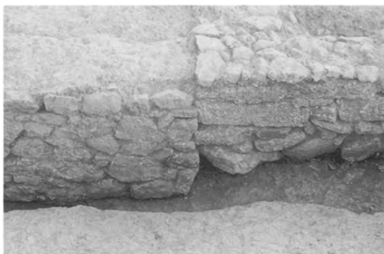
b. North walls of Buildings K-L:25-26 left, K-L:24-25 right (from north).
