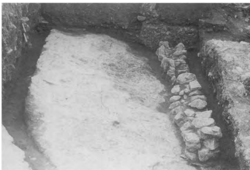
b. O:23, rock-cut drain, earliest wall (from east).
