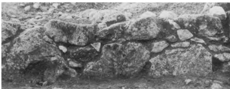
c. P:26, detail of Wall 2 (from north).
