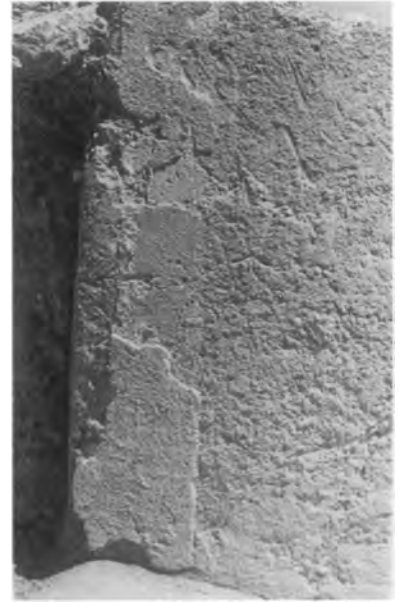
b. Building K-L:25-26, Room 2, east jamb (from south).
