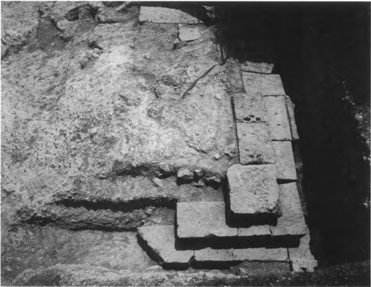
b. Building T-U:22 (from west).
