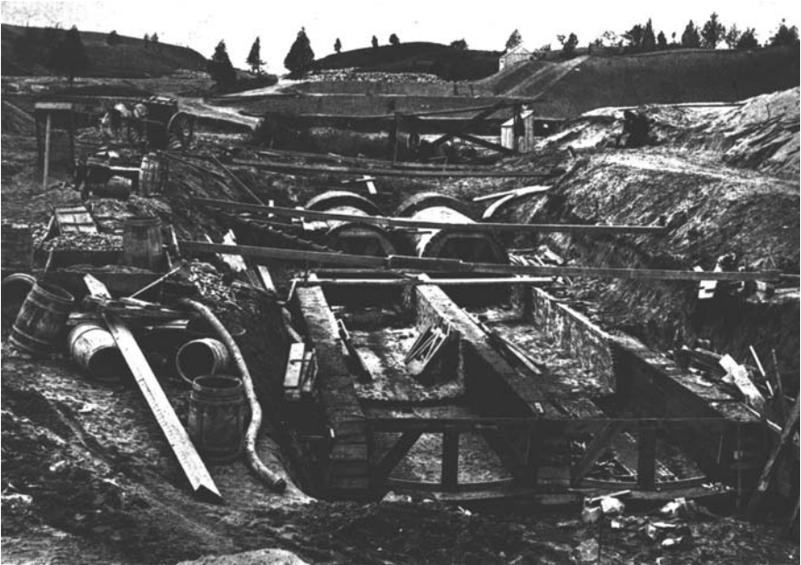
Fig. 5.5 Sewer construction at Field's Point. From the Annual Report of the City Engineer for 1891.
