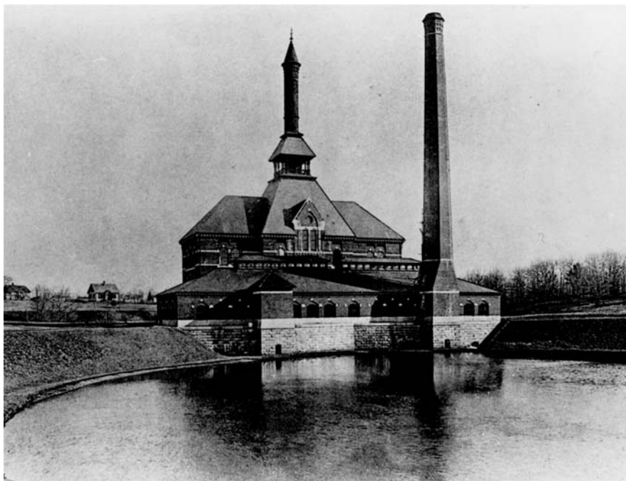
Fig. 5.3 The Pettaconsett pumping station on the Pawtuxet River for the Providence public water supply. From the Annual Report of the City Engineer for 1892.
