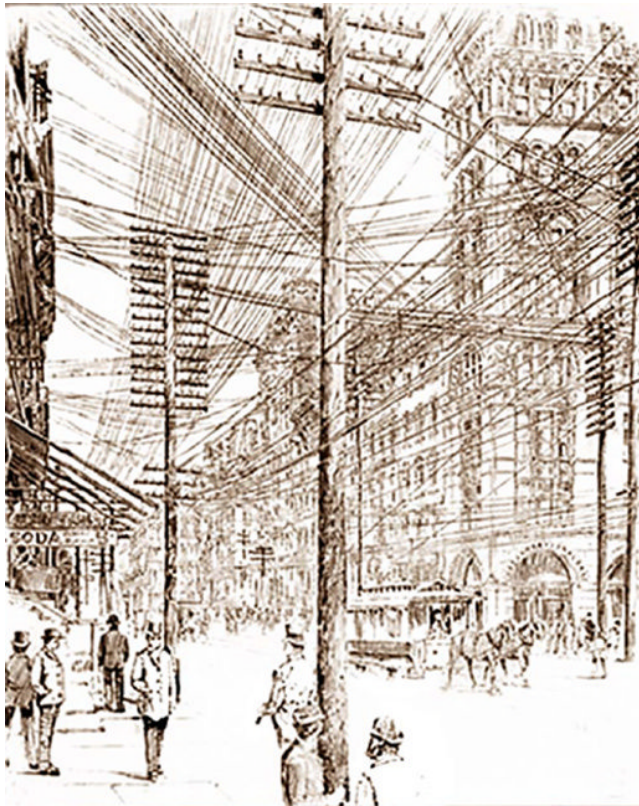
Figure 3.20 Overhead telephone and telegraph wires in Broadway, 1890. Source: Ref. [9]
