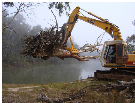
Figure 10.5 Re-snagging with large logs along the banks of the Murray River has favoured populations of native fishes such as Murray cod (Box 10.3). (Source: Martin Casey).
