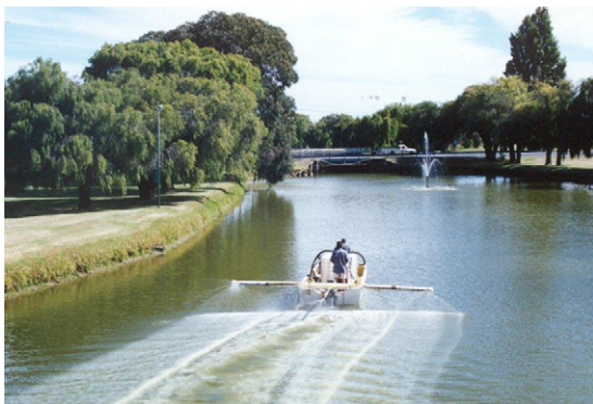
Figure 11.6 One management option for reducing eutrophication is to spray a phosphorus-binding agent into rivers. (Source: GeoCatch WA.)
