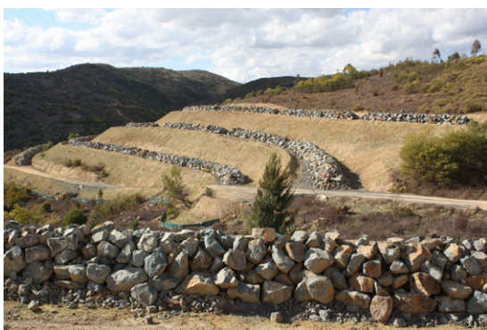
Figure 9.3 Rock-reef habitat created for Macquarie perch in the Cotter Reservoir, ACT, prior to enlargement and filling. (Source: Mark Lintermans.)
