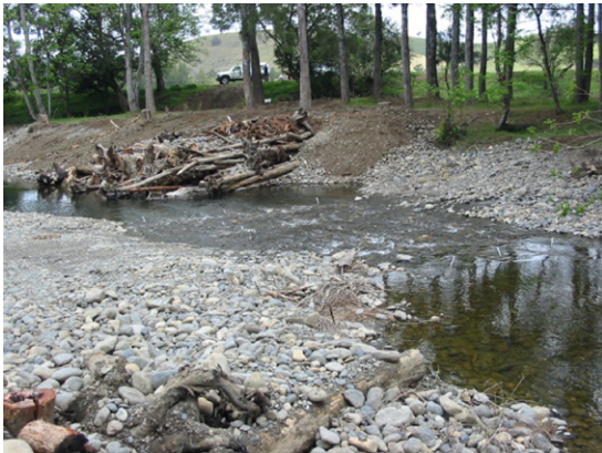
Figure 10.11 A newly built engineered log jam, upstream of Munni Bridge on the Williams River, NSW. These promote physical complexity of the channel and provide refuges from high flow. (Source: Sarah Mika.)
