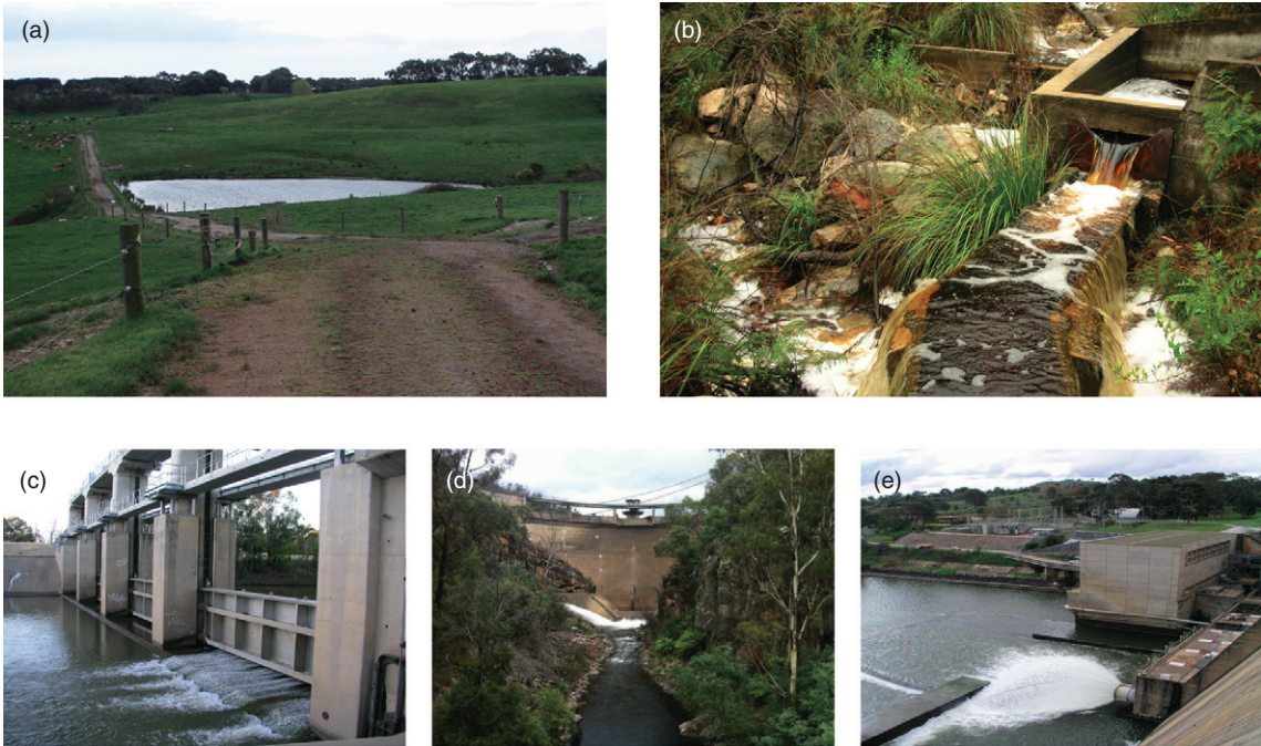
Figure 9.4 Diverse impoundments: (a) small farm dam on a headwater stream, (b) small weir, (c) large weir on the Gwydir River, NSW, (d) Bendora Dam on the Cotter River, ACT, (e) hydroelectricity generation outlet on the Hume Dam, NSW. (Source: (a) Ty Matthews; (b) Belinda Robson; (c), (d) and (e) Darren Ryder.)
