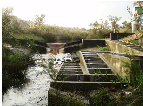
Figure 9.11 Fishway (right-hand side of photo) installed in the Goodga River, WA, to increase the area of breeding habitat available to a population of the western spotted galaxias Galaxias truttaceus hesperius , which is critically endangered. (Source: Stephen Beatty.)
