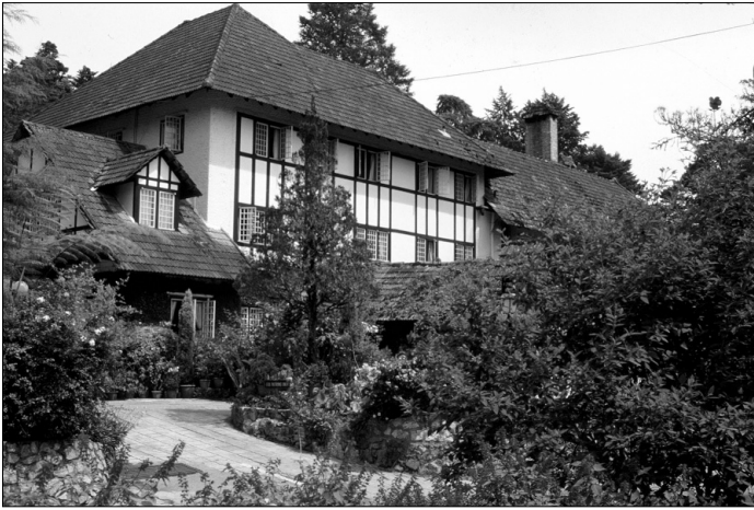
Figure 8.4 Cameron Highlands, Malaysia: Smokehouse Hotel. 1930s British hill-station architecture (2005)
