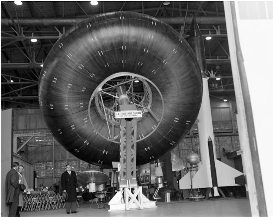
**Fig. 5.8** Prototype of an inflatable space station concept with a solar power system collector from 1961 (NASA)
