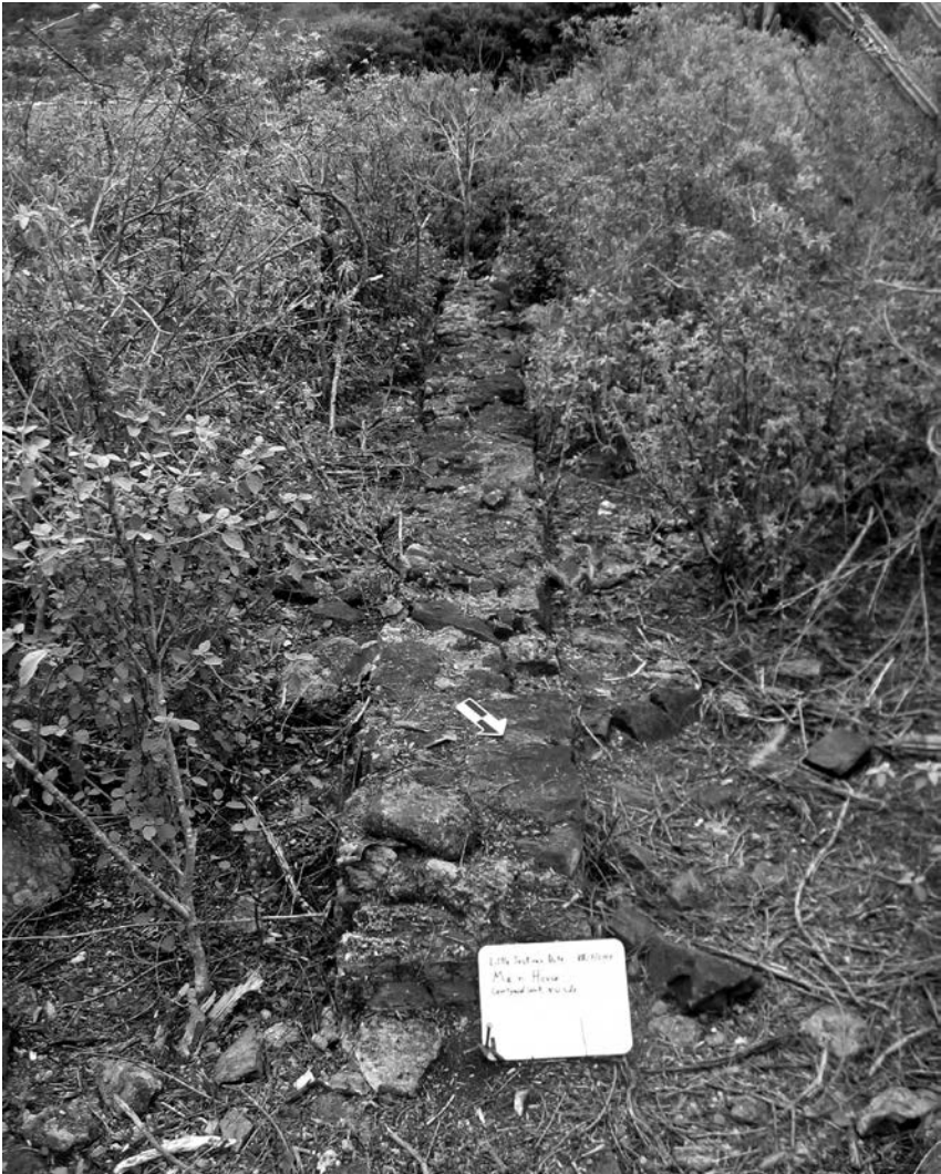
Figure 2.8. Rear (northwest) wall of the Lettsom house, nearly level with the slope, facing southwest.
